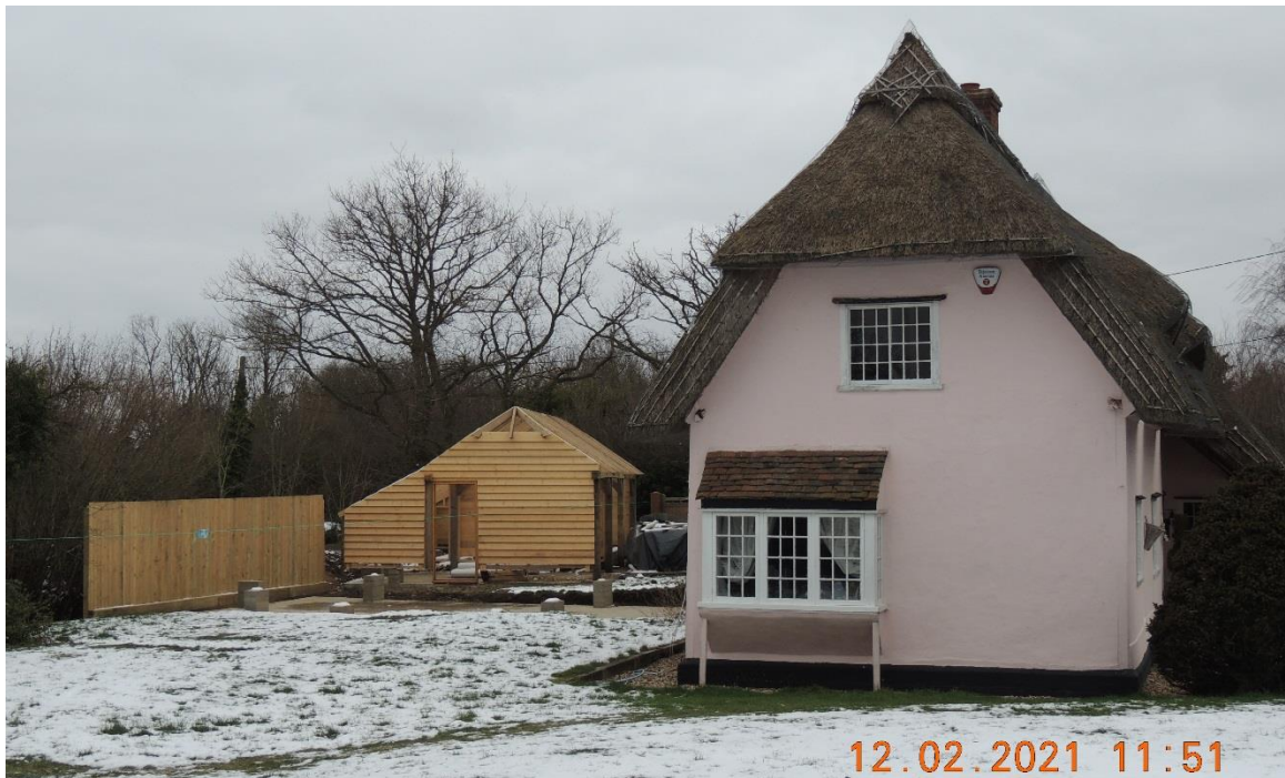
Photo 3: Pheasant Cottage – Side/End Elevation (looking north-east)
