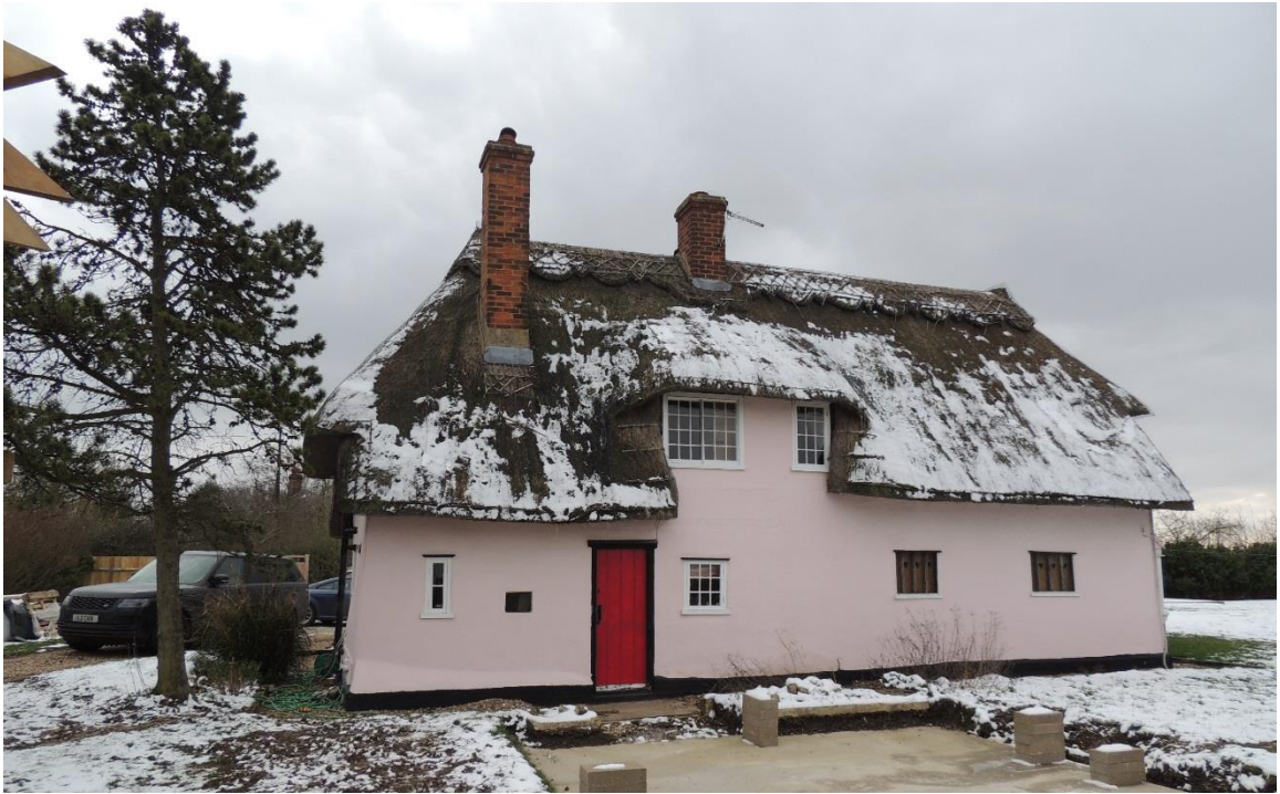
Photo 1: Pheasant Cottage – Rear Elevation (looking south-east)
