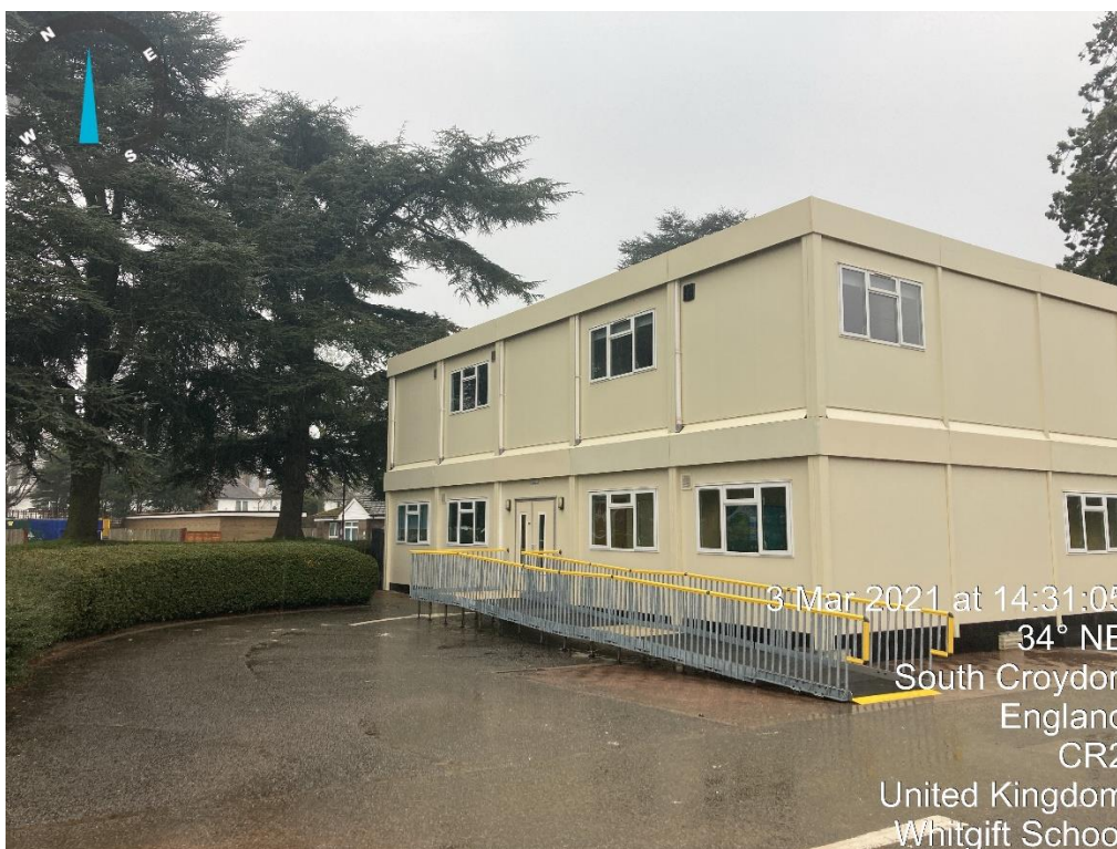
Plate 8. View north-east from main school building of Classroom CSA with temporary classrooms built on pre-existing hardstanding
