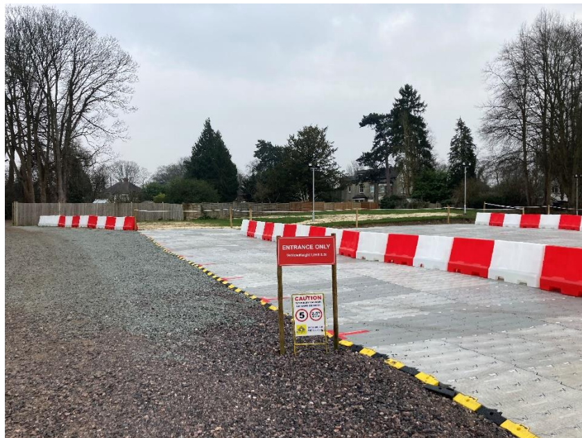
Plate 4. Supa-Trac on pre-existing hardstanding facing east.
