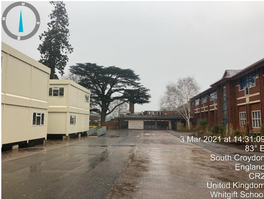
Plate 9. East facing view of Portakabin classrooms screened by the main school building.
