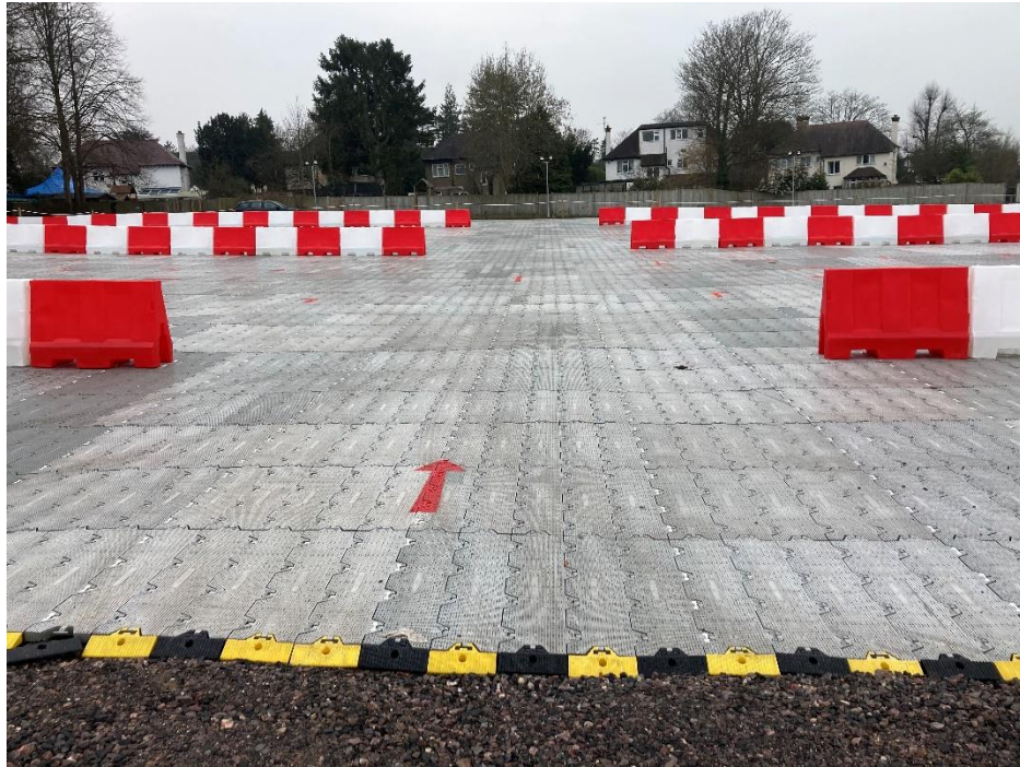
Plate 5. Supa-Trac on pre-existing hardstanding facing south
