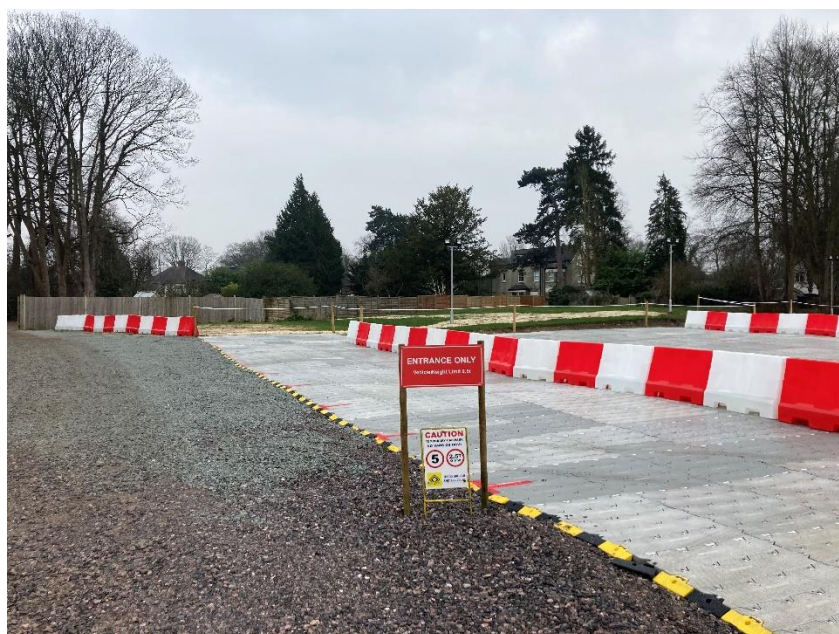
Plate 2. Supa-Trac on pre-existing hardstanding facing east.
