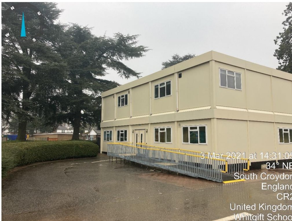
Plate 6. View north-east from main school building of temporary classrooms built on pre-existing hardstanding
