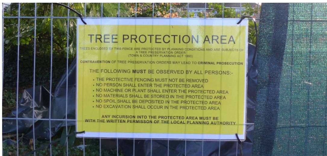
Protective fencing in accordance with B.S. 5837
