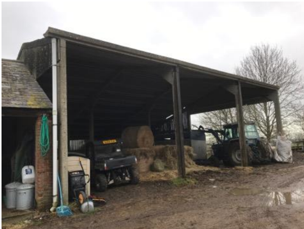
Photo 3: East elevation of Building B1
