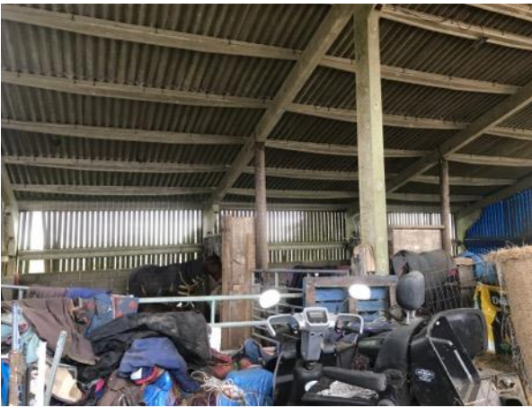
Photo 9: Interior of Building B1
