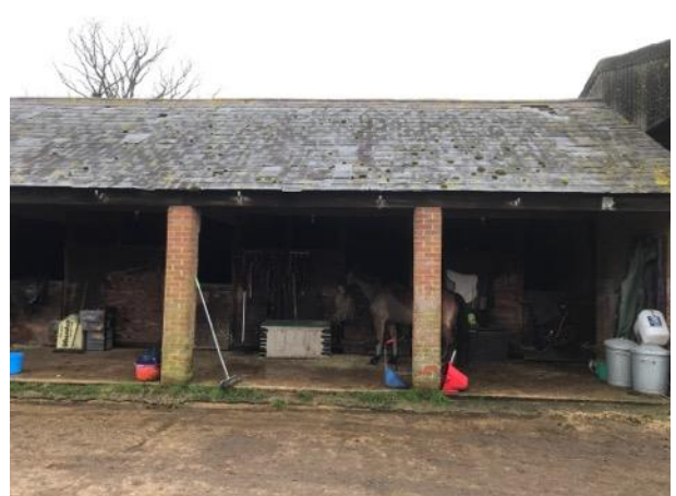
Photo 4: East elevation of Building B2
