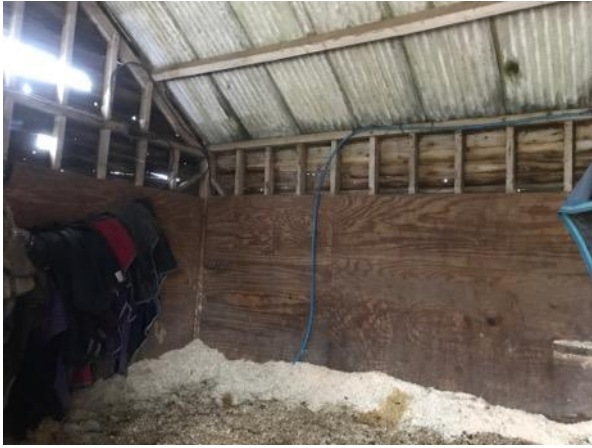
Photo 7: Interior of Building B3
