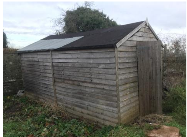
Photo 6: South east elevation of Building B4
