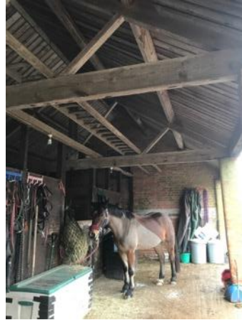
Photo 8: Interior of Building B2
