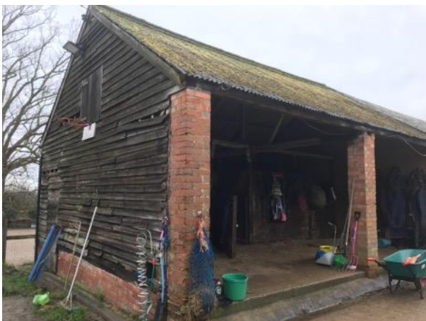
Photo 5: South east elevation of Building B3
