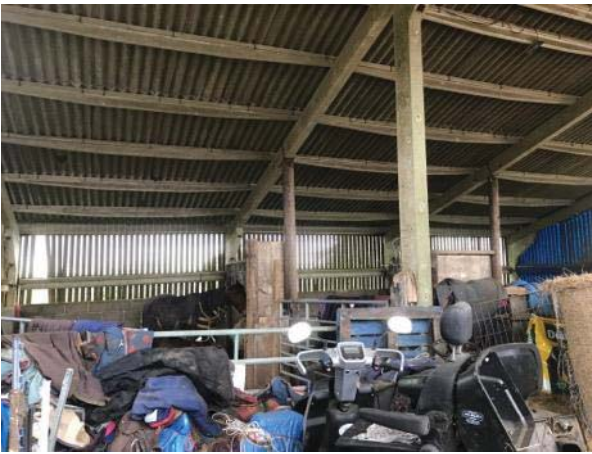
Photo 9: Interior of Building B1
