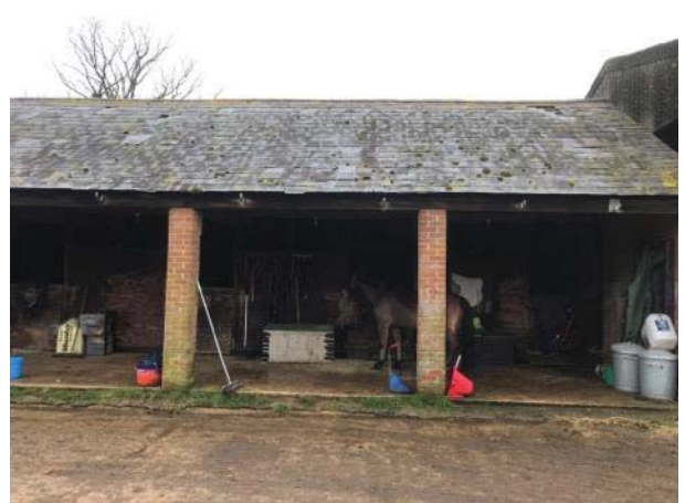
Photo 4: East elevation of Building B2
