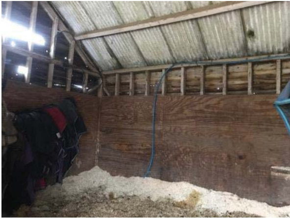
Photo 7: Interior of Building B3
