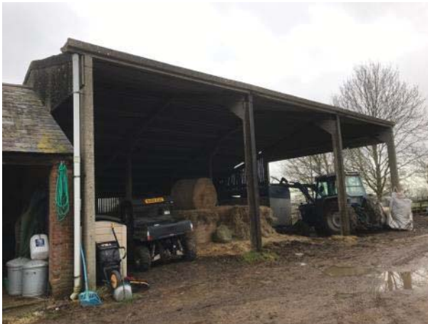
Photo 3: East elevation of Building B1
