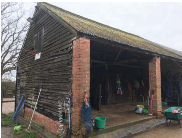
Photo 5: South east elevation of Building B3
