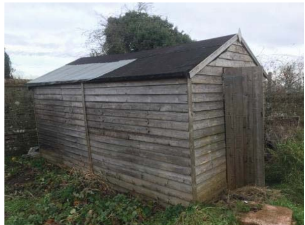
Photo 6: South east elevation of Building B4
