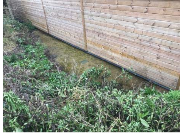
Photo 14: Waterbody TN2 – standing water north east of the site
