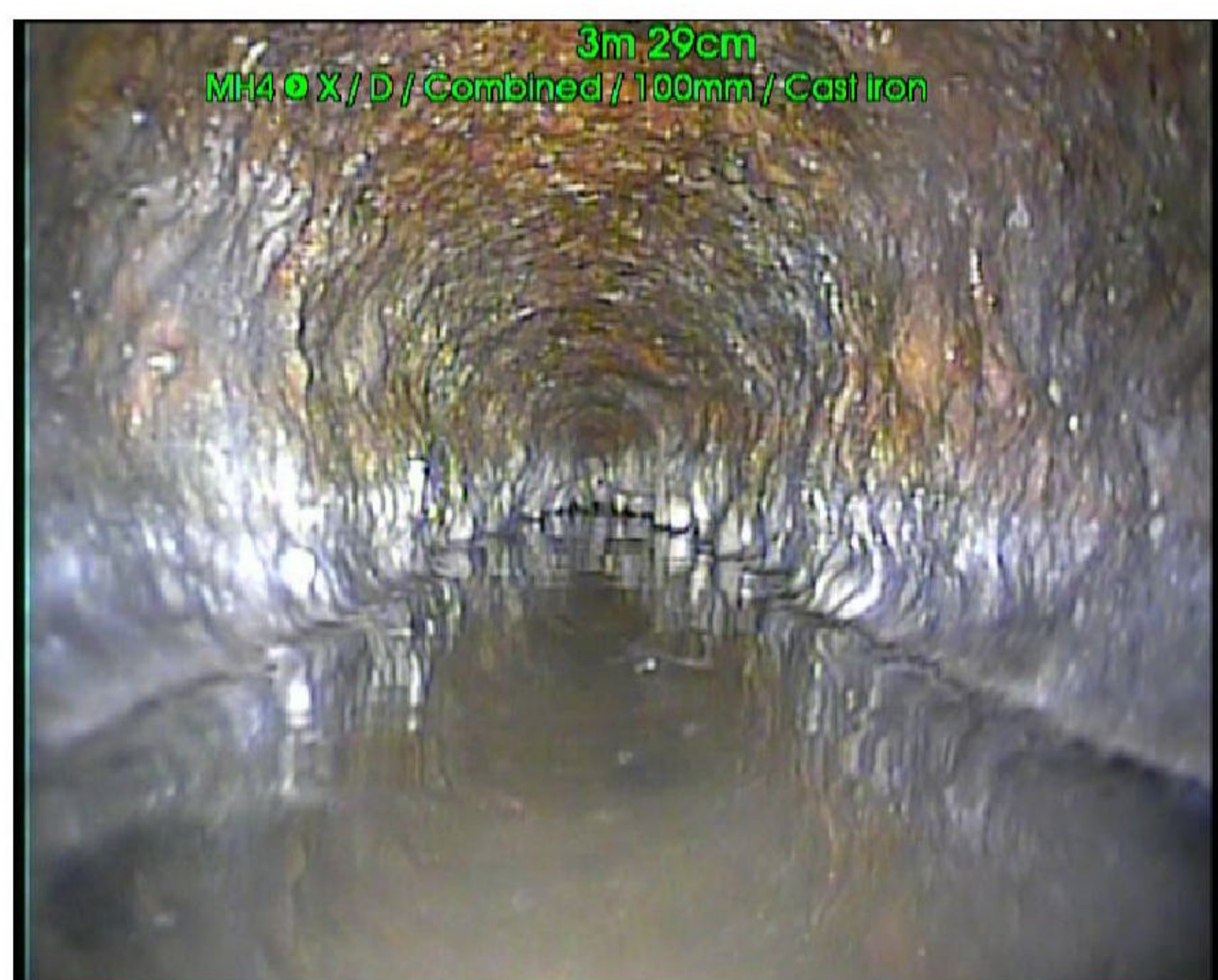
Photo: 9_9_44_A.jpg 3.2m, Water level 10 % of the vertical dimension
