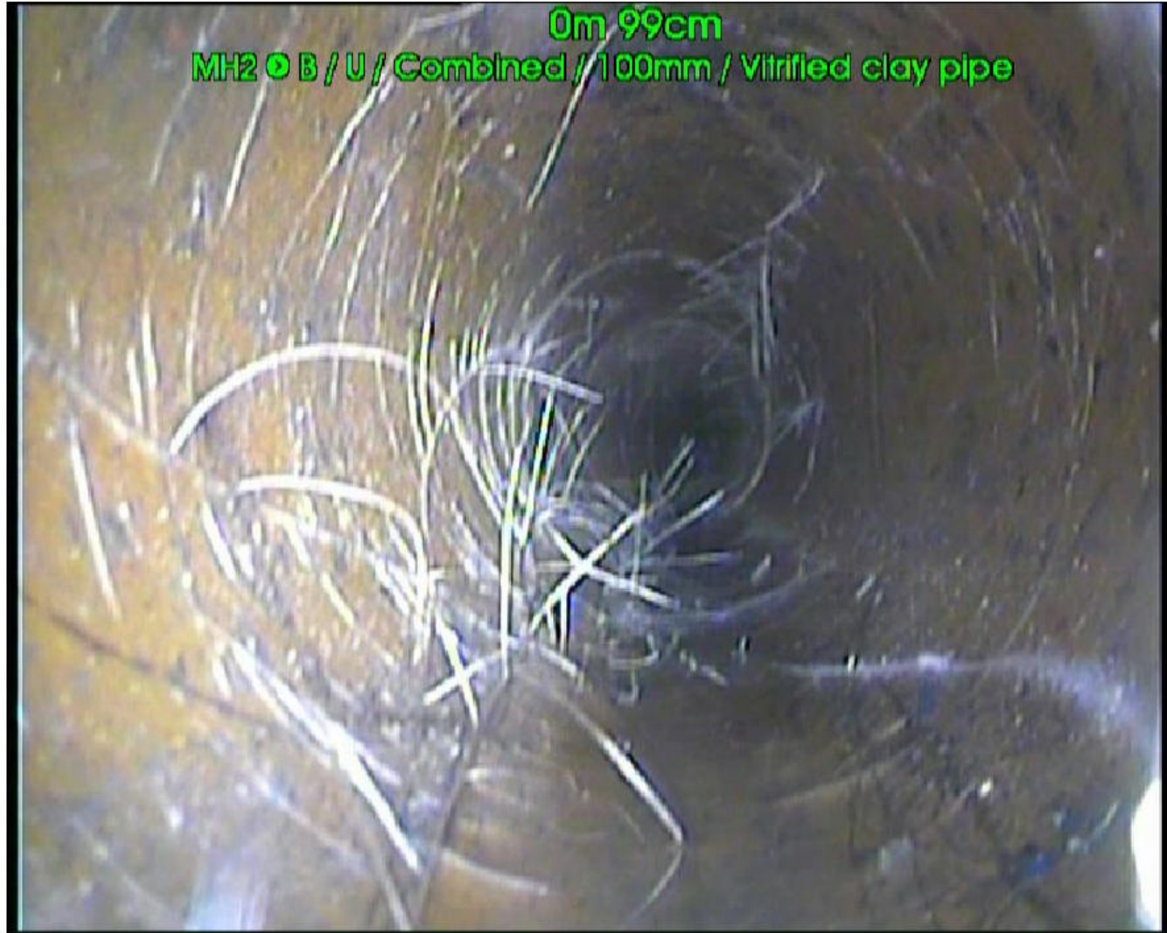
Photo: 5_5_18_A.jpg 0.99m, Roots, fine S1
