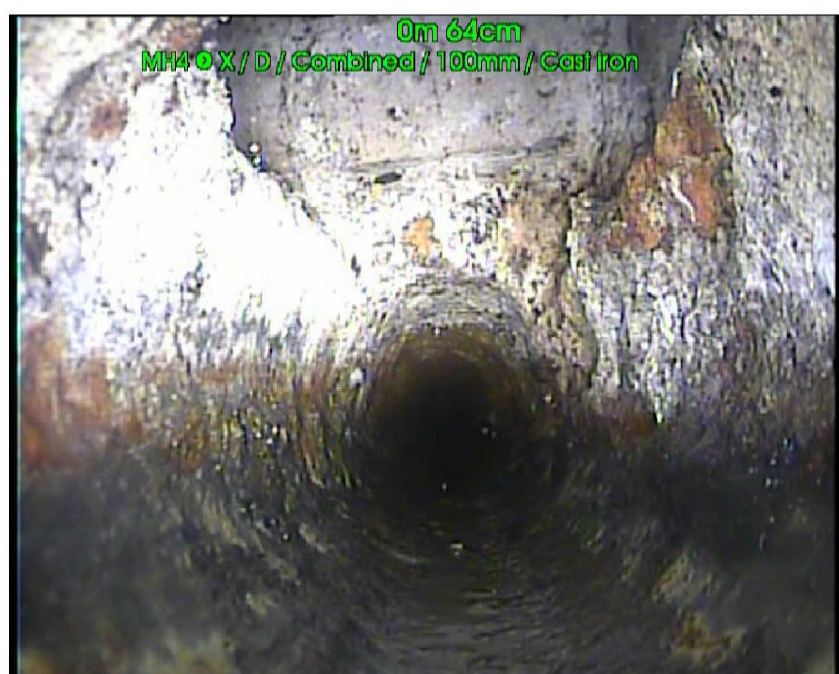
Photo: 9_9_40_A.jpg 0.6m, General remark POSS HOLE OR CONNECTION
