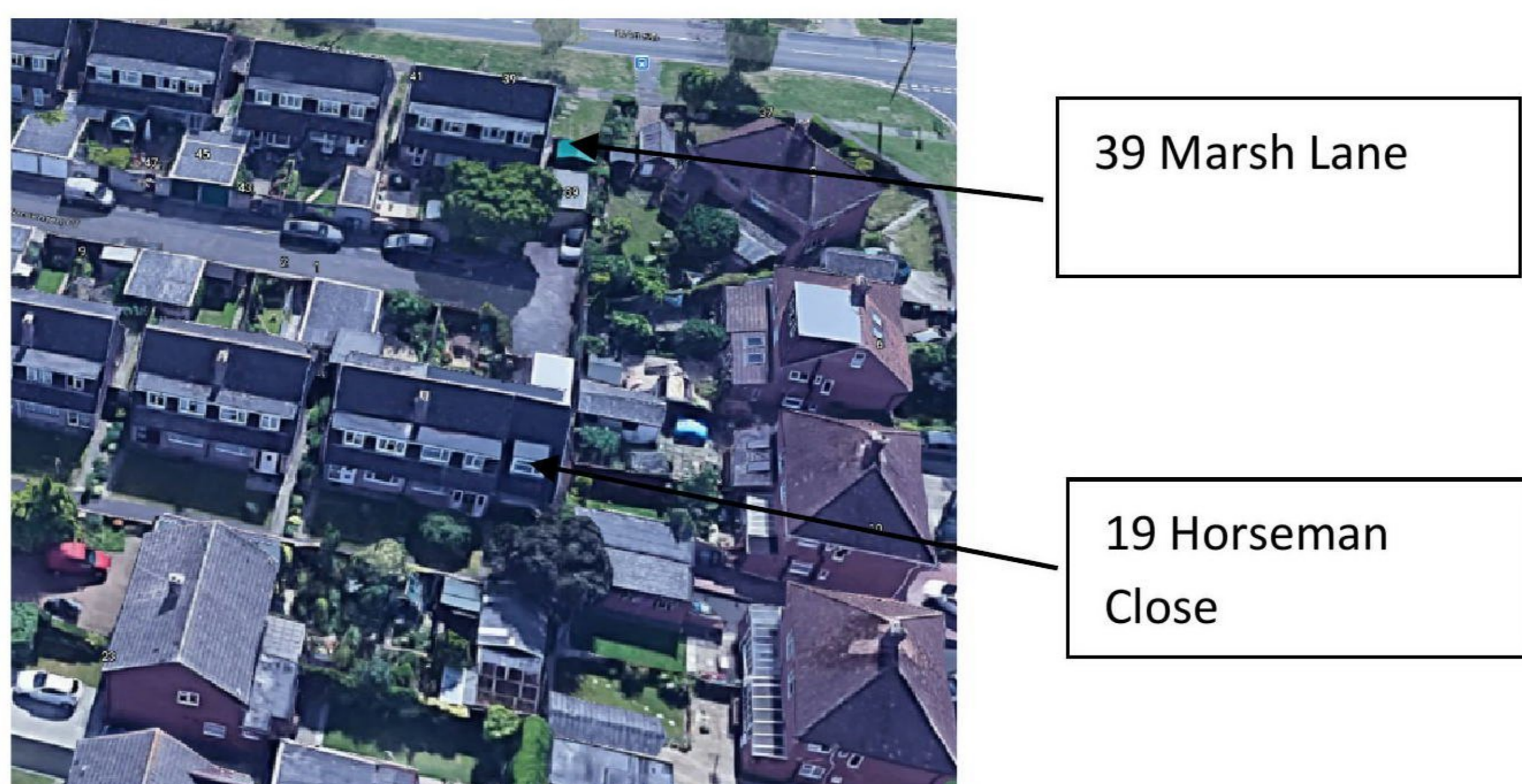
Figure 3 - Areal View of no 19 Horseman Close
