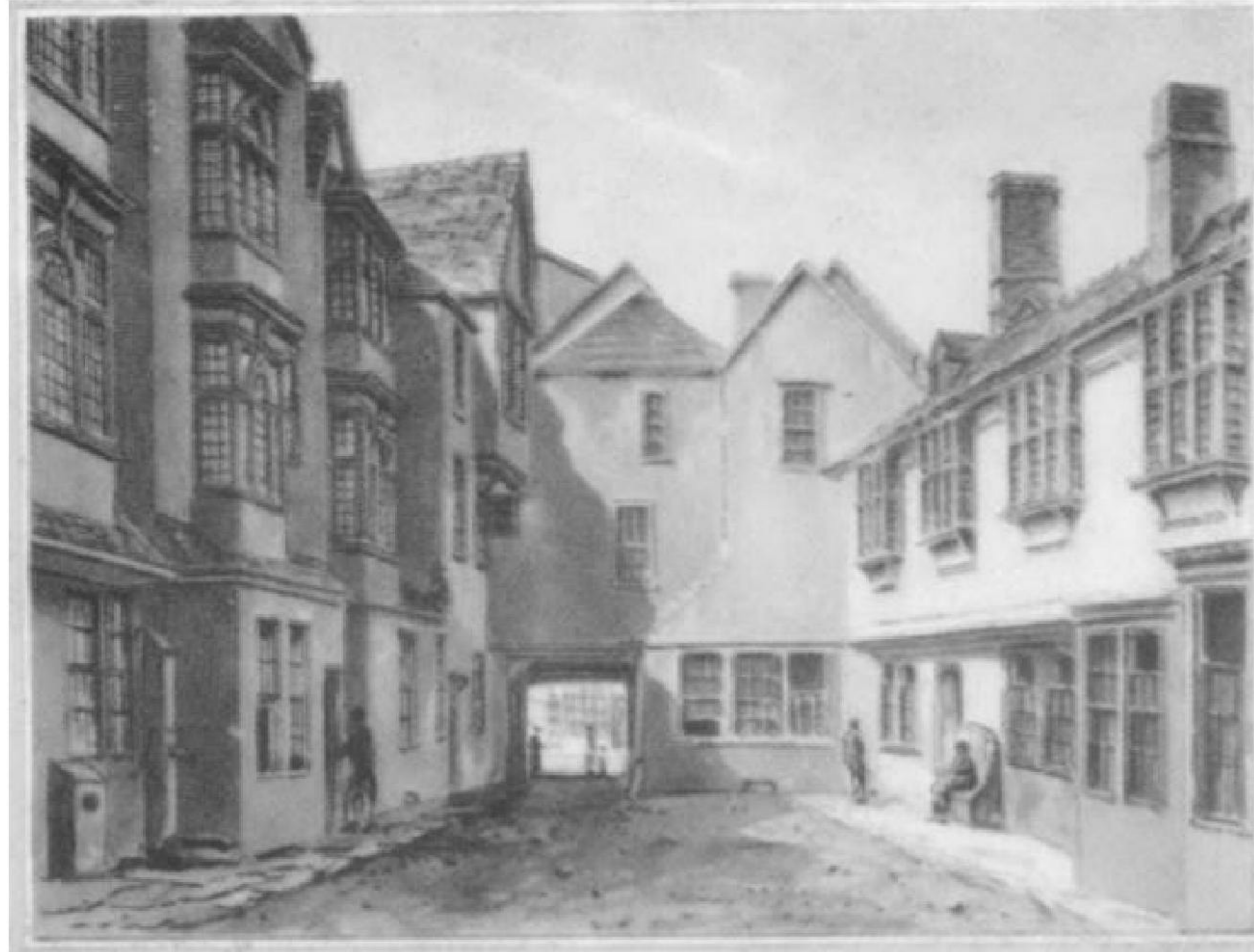
A sketch by Buckler in 1824 shows the Golden Cross courtyard, looking towards the passageway off Cornmarket Street. On the left-hand side, the bay windows survive as shown. The structure over the passageway has been rebuilt, although the right-hand gable end survives as shown. Prior to its rebuilding, the rear portion of 4 Cornmarket Street appears to have had a jettied gable looking out onto the courtyard.
