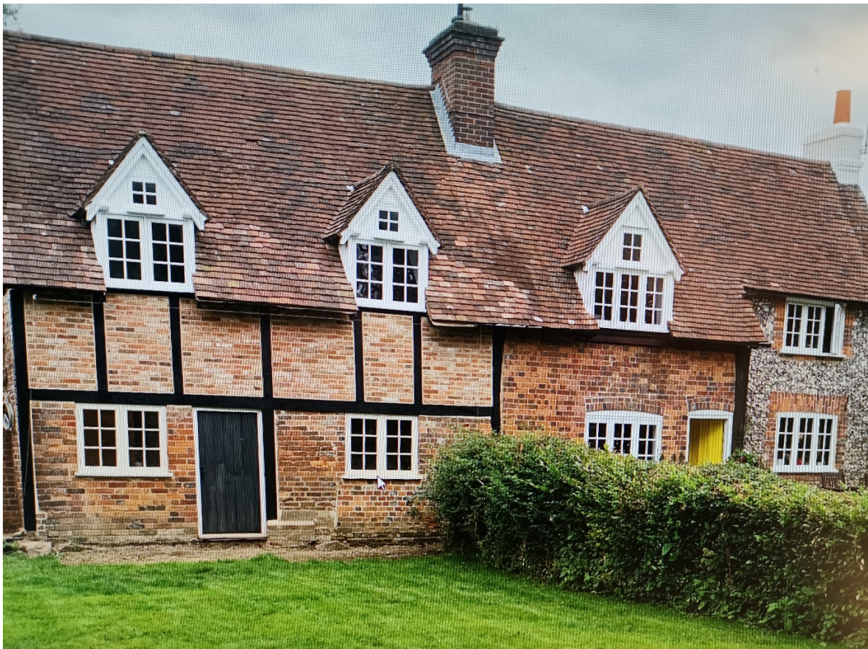
Renovated Front Elevation
