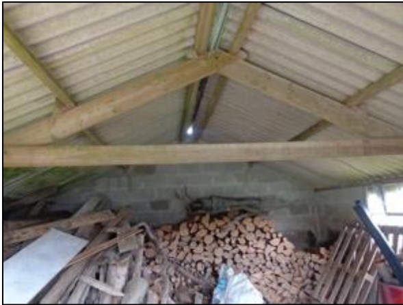
Figure 3. Interior view of barn
