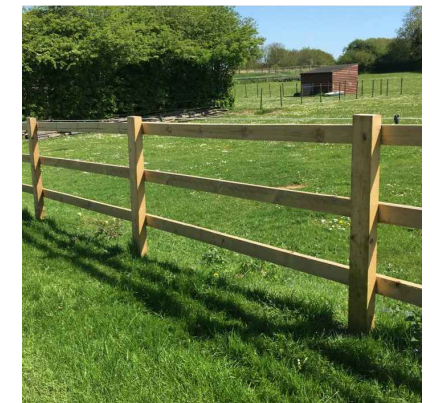
IMAGE OF TIMBER POST & RAIL FENCE
