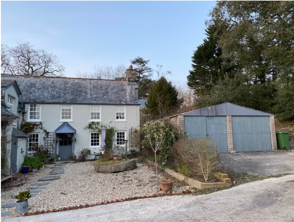
Photo showing South Elevation
