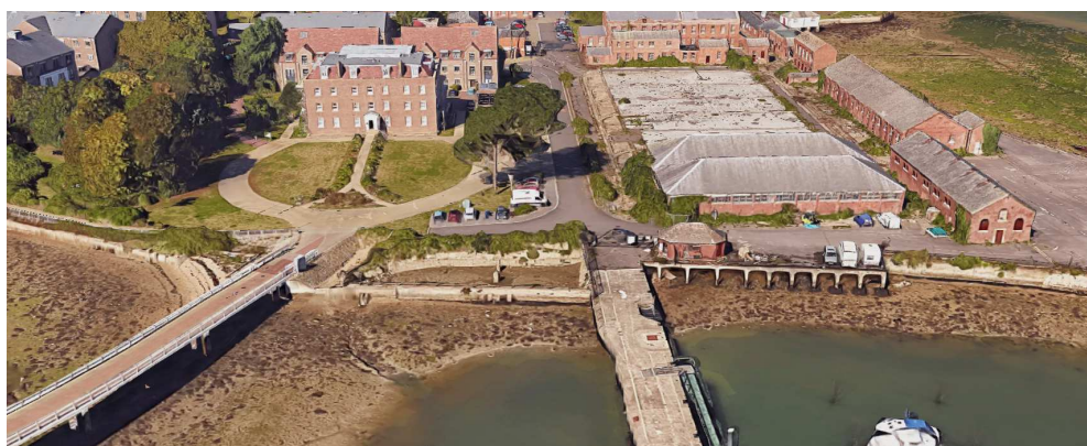
Figure 6 - View of Frontage E
