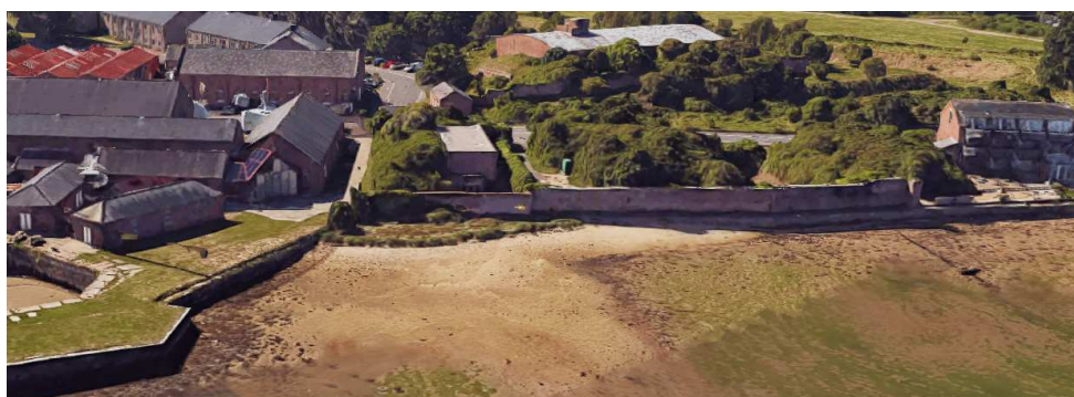
Figure 4 – View of Frontage A
