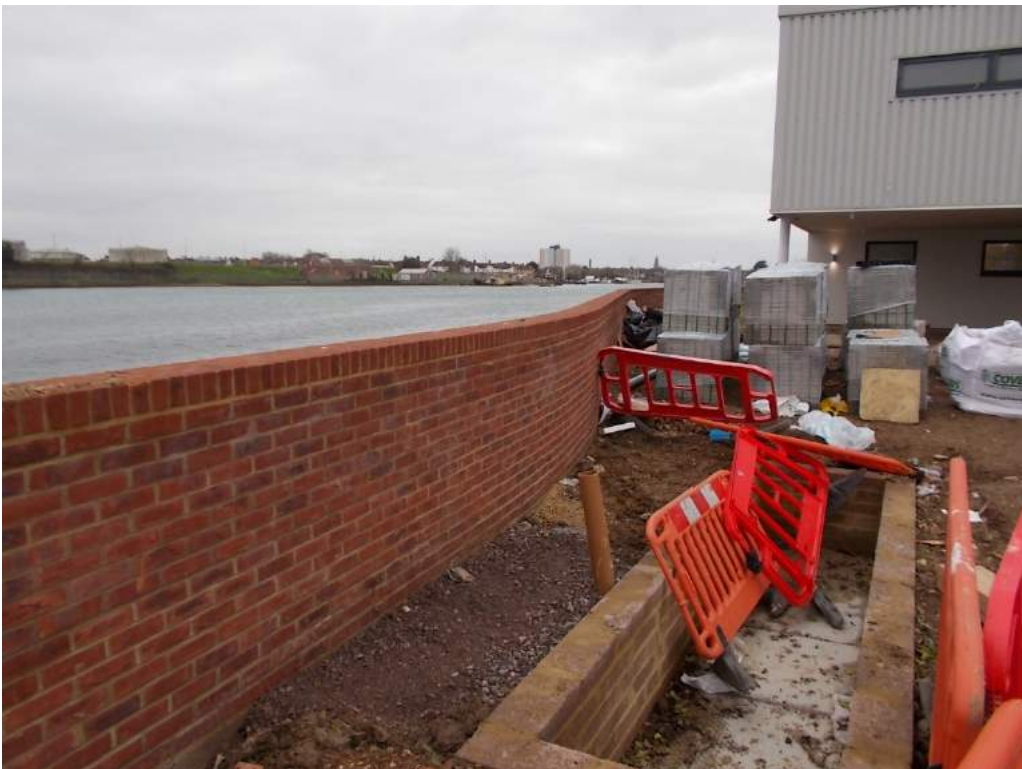
Existing sea wall at shell filling rooms
