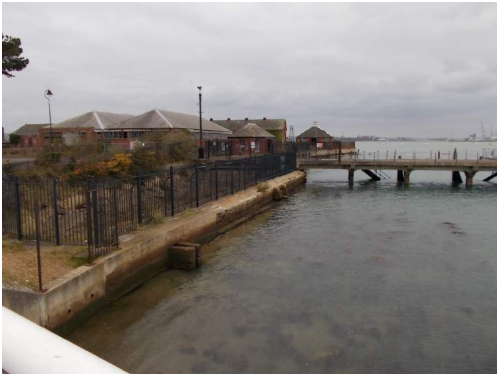
Existing defences South of site to East of Heritage Way
