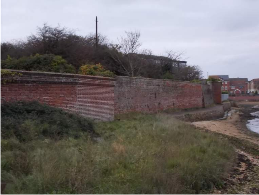
Existing seawall adjacent C Magazine building
