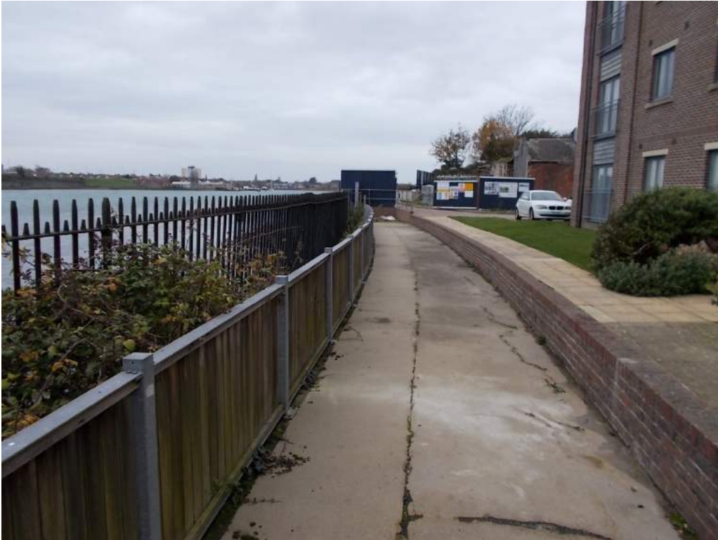
Existing landward flood wall at Searle Drive
