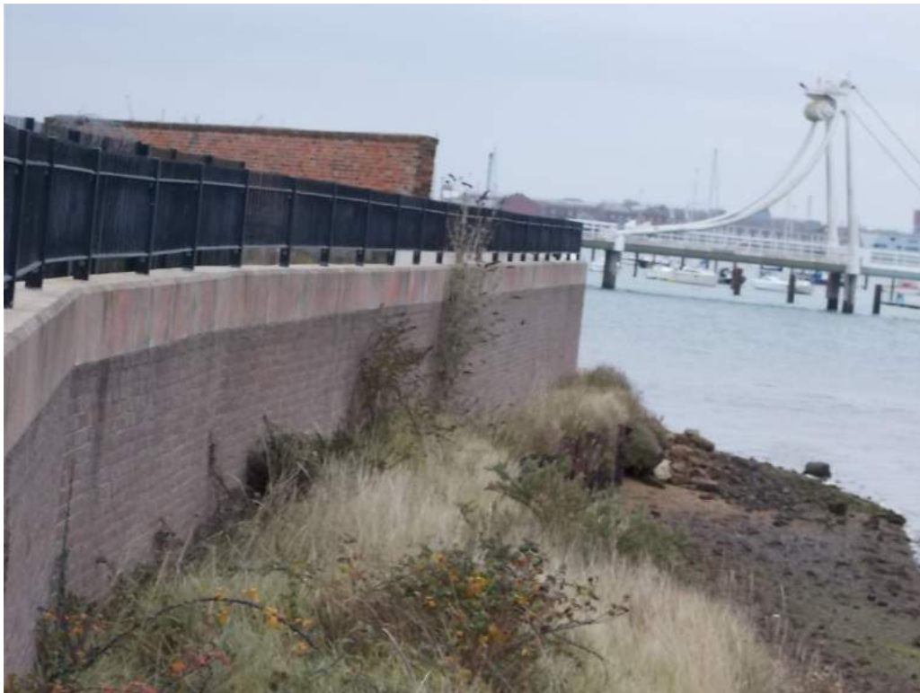
Existing seawall to Shell Filling Rooms west of the site
