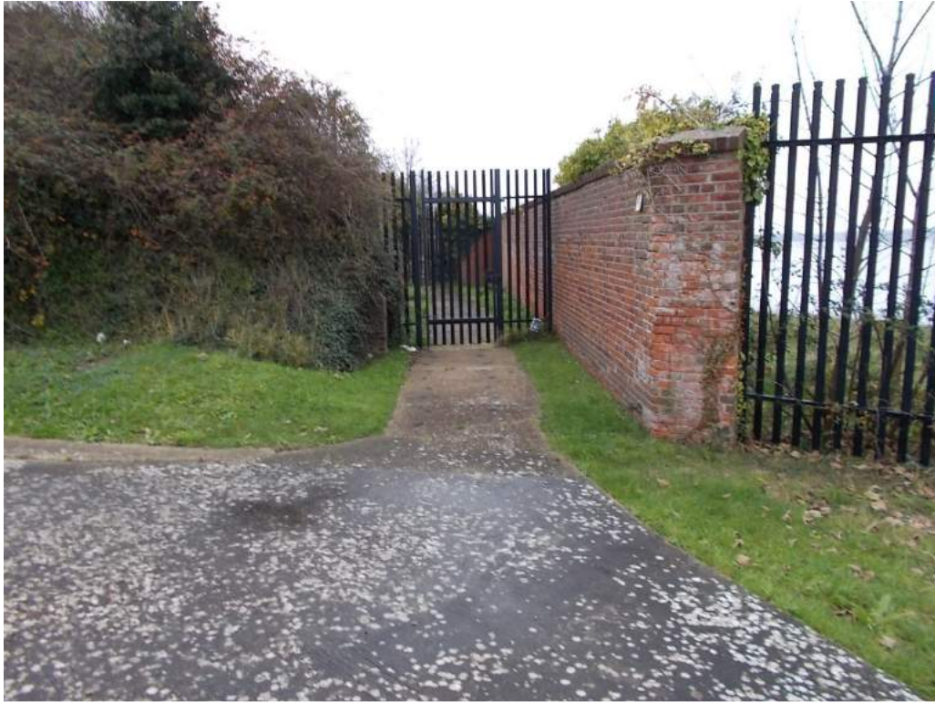
Existing Seawall North of site
