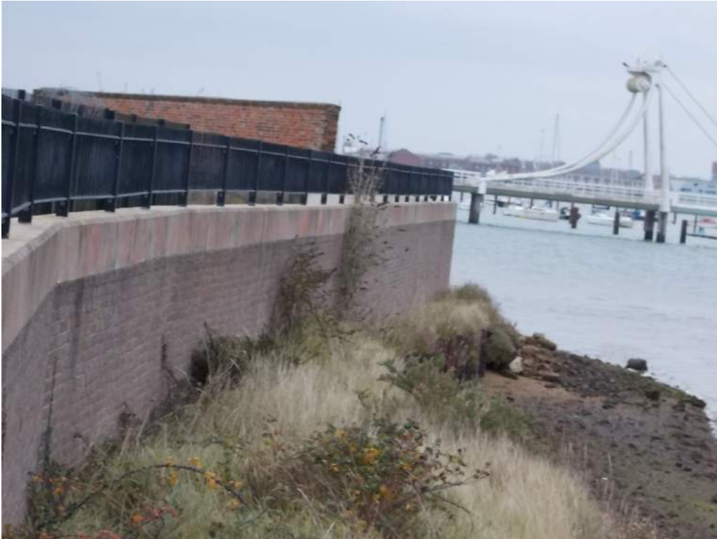
Existing sea wall on approach to shell filling rooms
