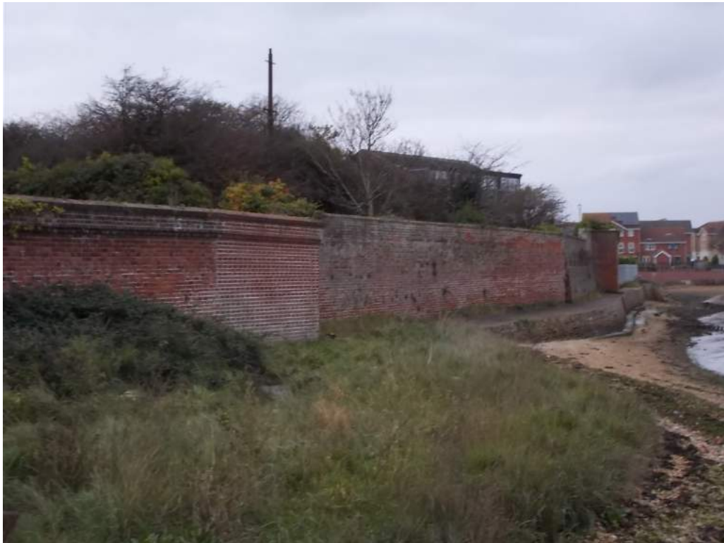
Existing Seawall North of Site
