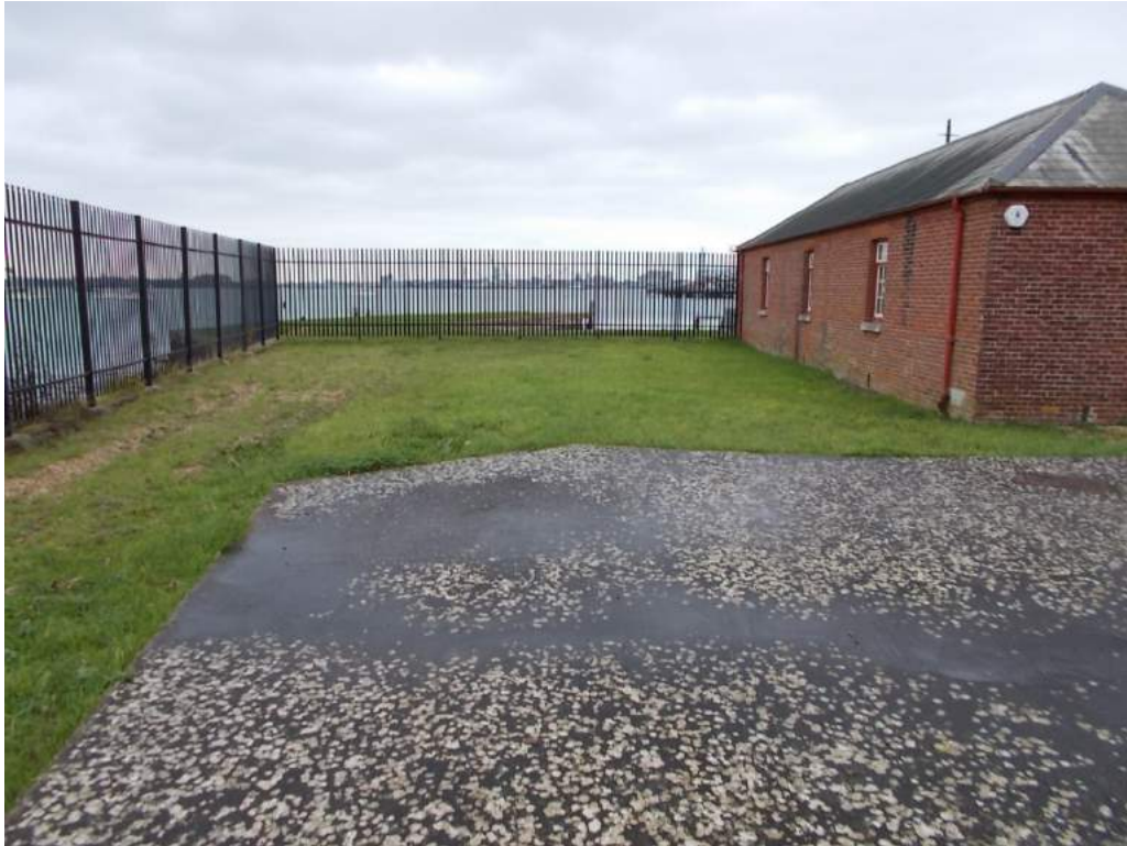
Building U2 site and north elevation Building U
