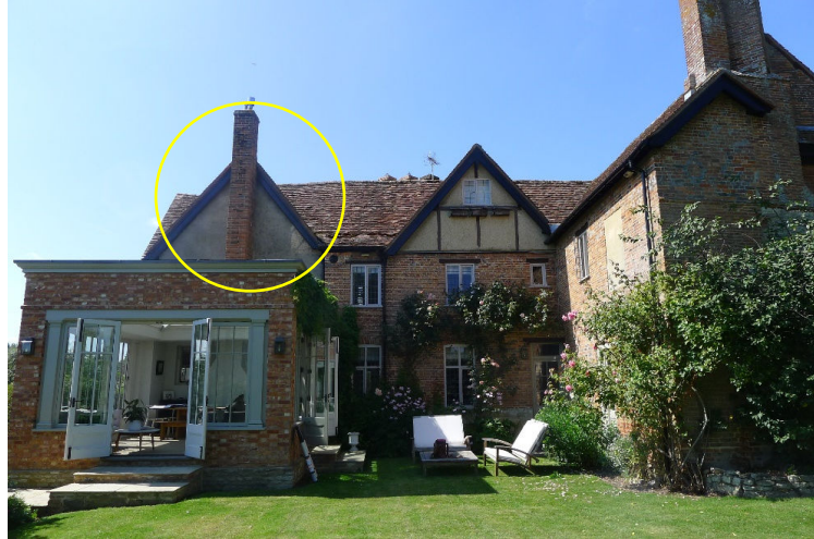
Fig 1: View of the east facing elevation
