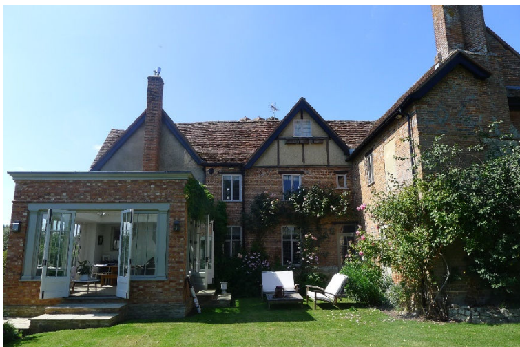
Fig 1 [left]: View of the east elevation
