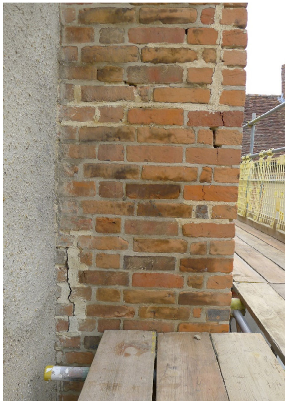
Fig 4: Detail of south elevation of the stack
