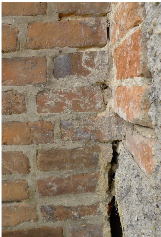
Fig 6: Detail north of stack - tothing detail with gable
