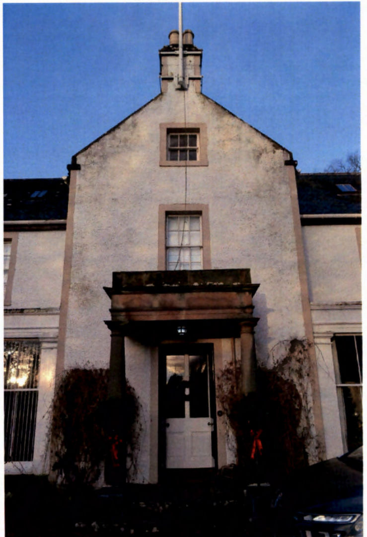
Entrance to Wardlaw House
