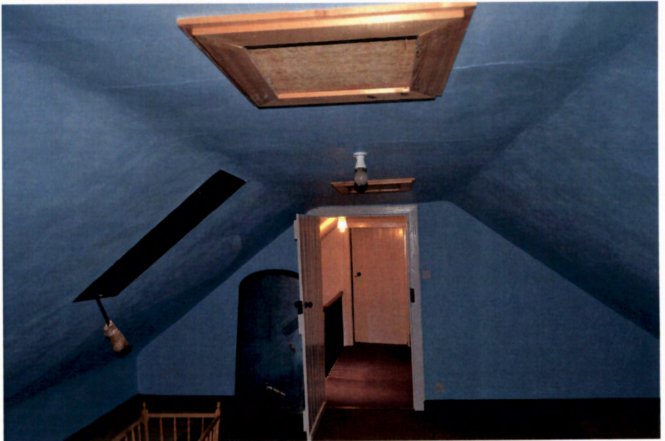
Photo of existing Second floor Attic Bedroom 7 with Landing beyond
