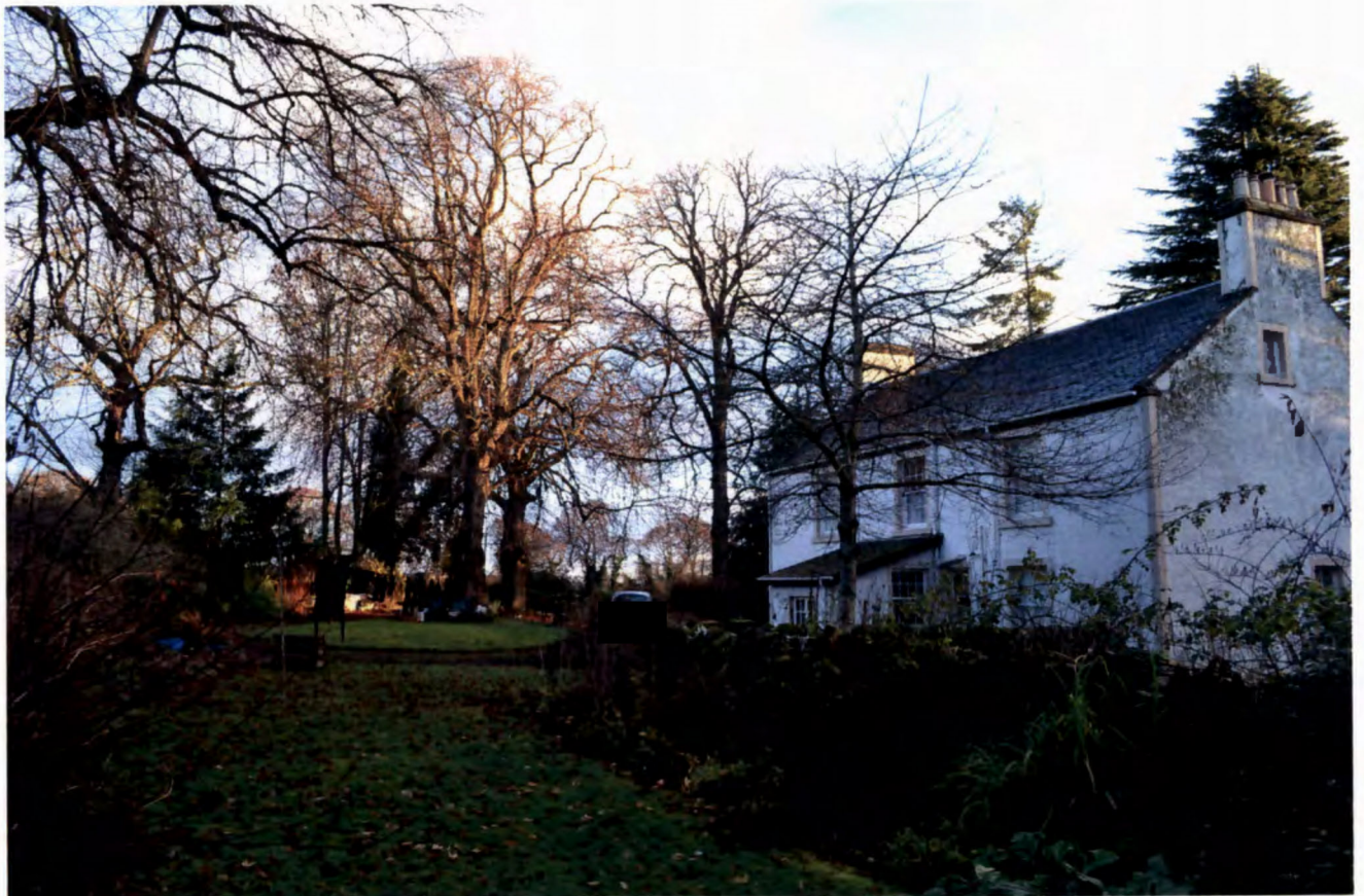
Photo of the rear of Wardlaw House
