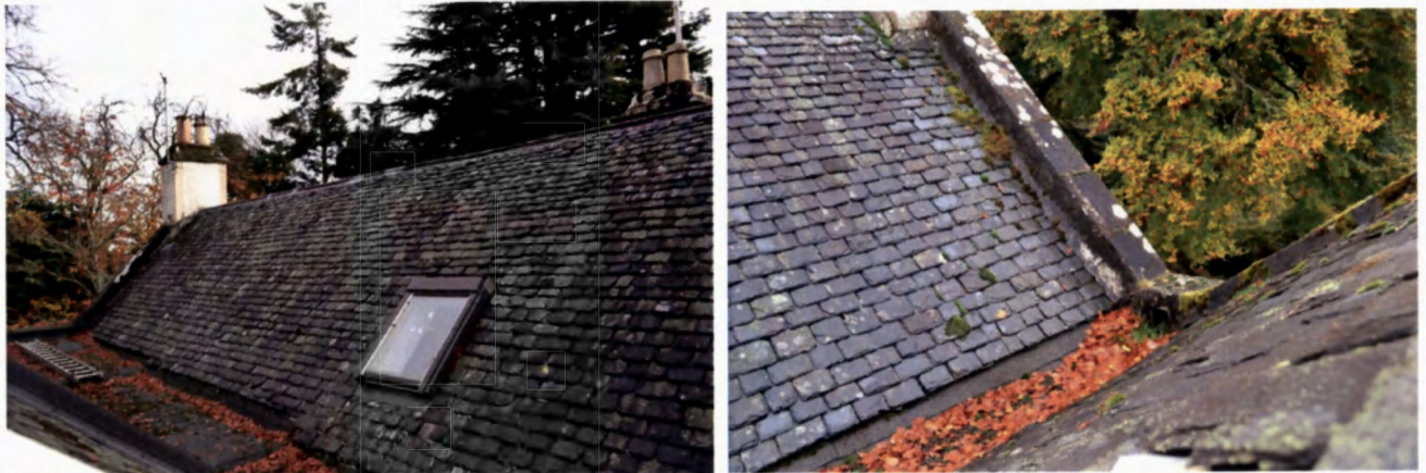
Photos of Valley Gutter “Wide” end + “Funnel” end
