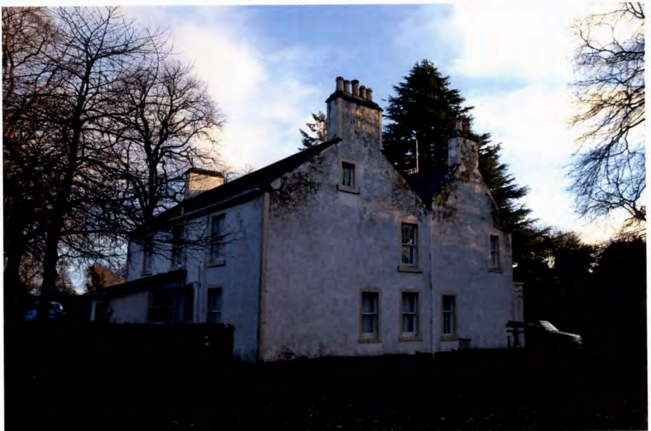
Photo of 2021 West Side Elevation to garden showing removal of Greenhouse + Doorway converted to window
