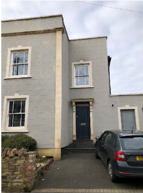
Image 1: View from front of property - solar panels not visible from road
