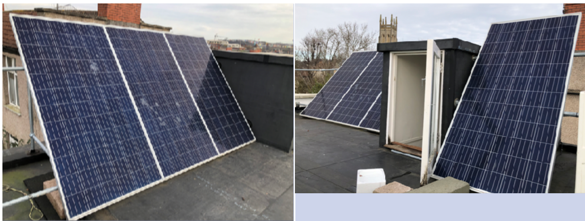
Image 4 & 5: Views of solar panels from the roof
