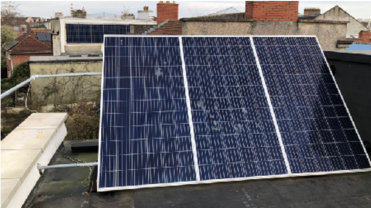
Image 4: Views of solar panels from the roof
