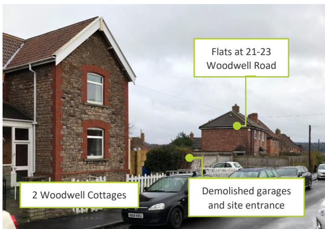
Image 5: Woodwell Road, 2 Woodwell Cottages, the now demolished garages and proposed entrance
