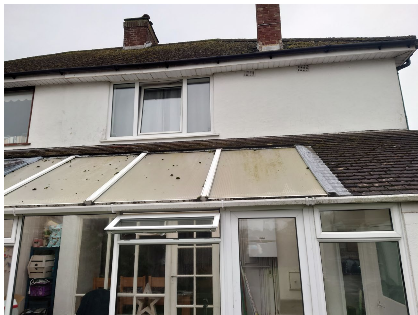
5: View of existing roof at rear (North) of property
