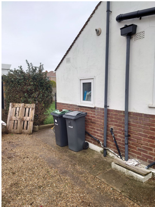
2: View of rear corner (West) of property
