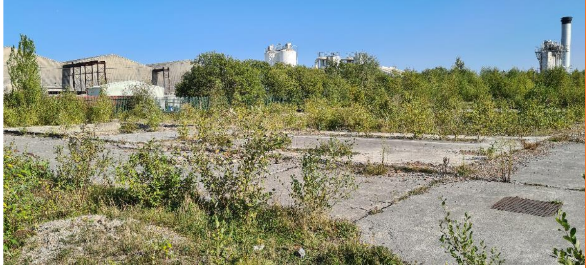
PLATE 1 VIEW LOOKING EAST
