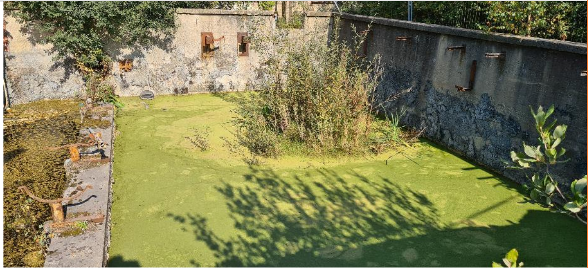
PLATE 2 VIEW OF WATER FILLED PIT IN NORTHEAST
