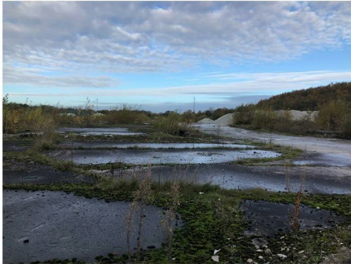
PLATE 1 SHOWING AREA OF HARDSTANDING
