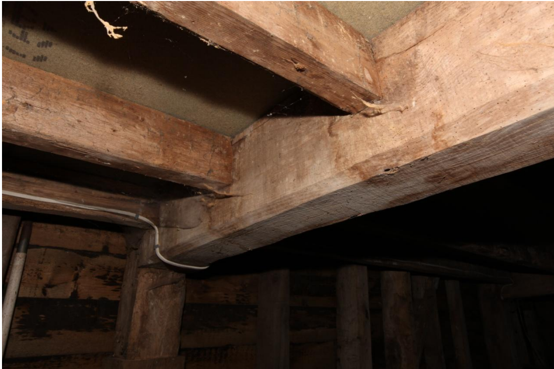
Illus. 9. A detail from the north-east of the neatly chamfered principal joist between bays B & C showing the tall-sectioned common joists which are of plain pine and typical of those elsewhere in the ceiling.
