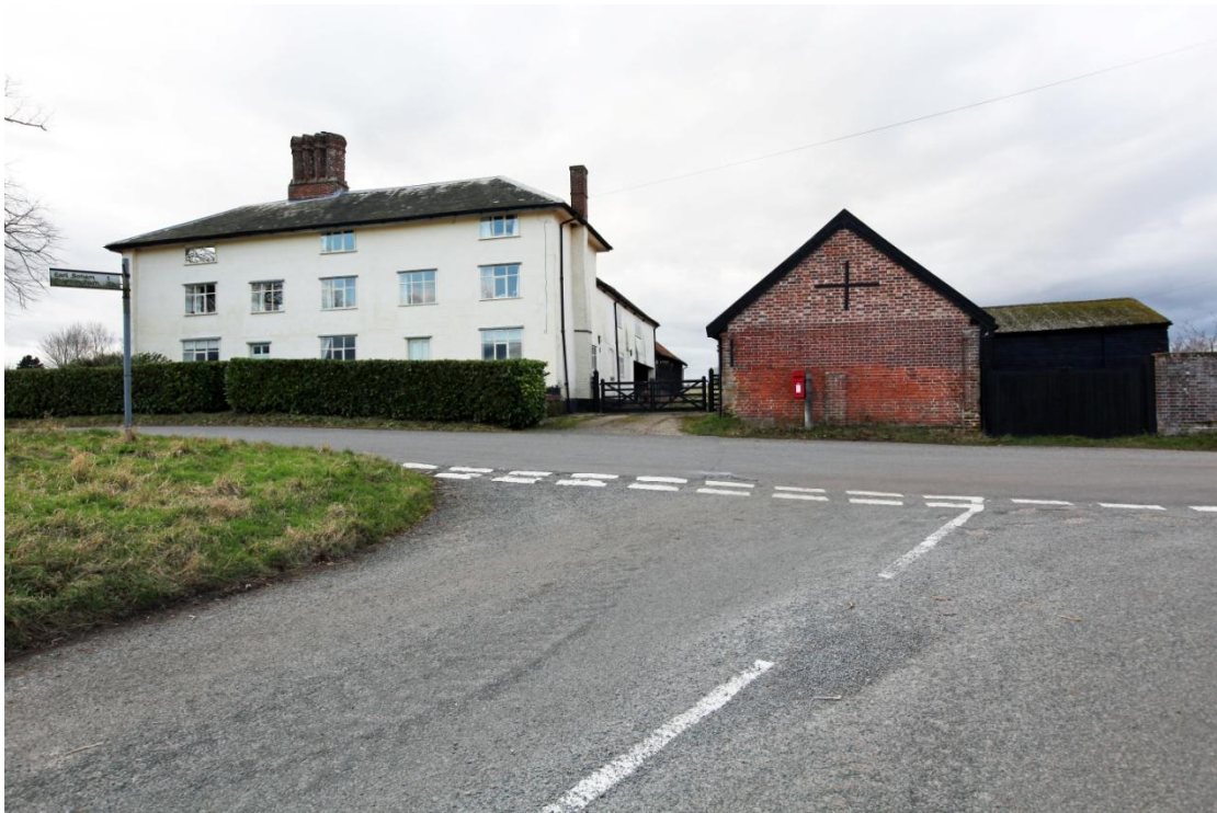
Illus. 1. Ashfield Lodge from Low Road to the north-east showing the extent to which the property dominates the junction. The walls of the original 16 th century farmhouse rose only to the lintels of the first-floor windows but were raised in the 19 th century. The rear barn is visible between the house and the mid-19 th century shelter-shed on the right.
