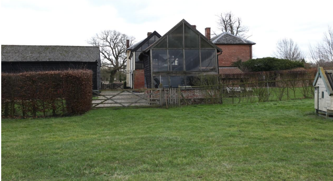
Illus. 3. The site from the west showing the rear barn's bowed northern wall with the threshing barn on the left. The former's western gable was completely rebuilt and glazed in the late-20 th century retaining only its brick plinth. The northern wing of the house was glazed in the same manner on its upper storey.
