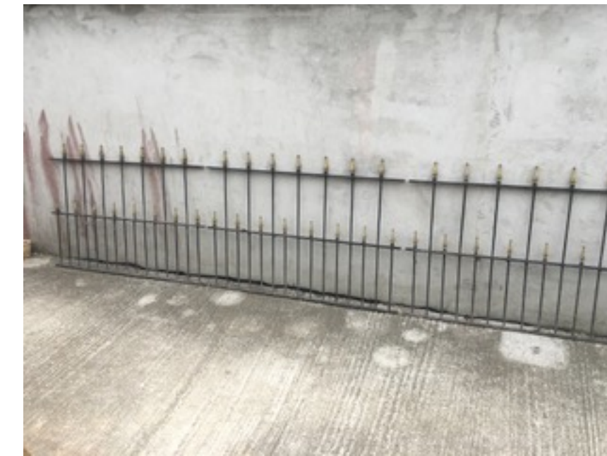
image of railings to be fitted after refurbishment & painted
