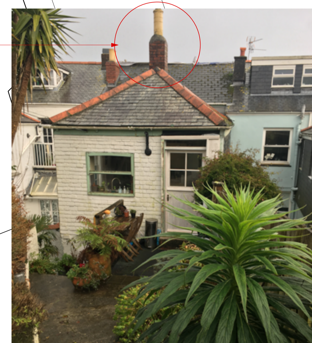
rear elevation showing chimney to be removed
