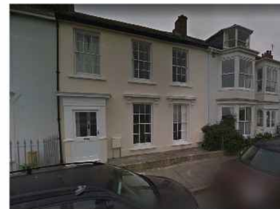
street view showing railings to adjoining properties but non to No.22
