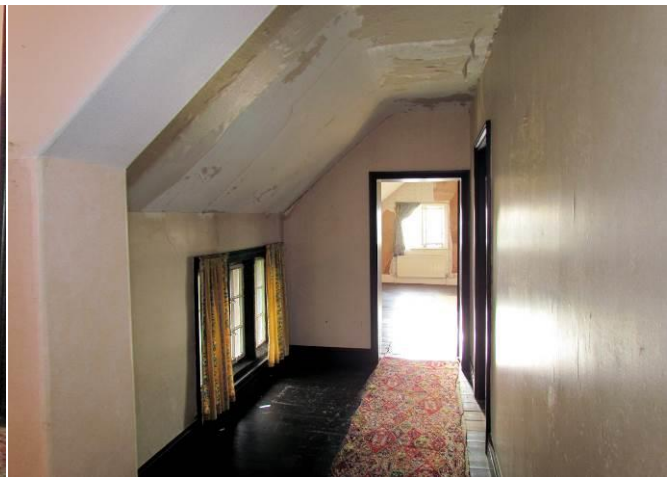
First Floor Corridor
