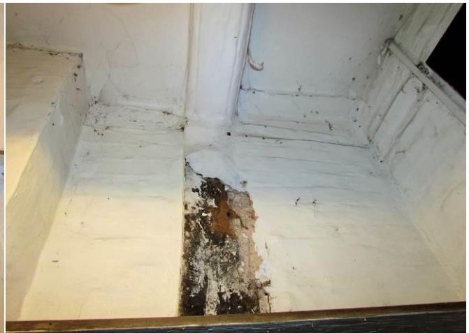
Timber Framing and Beam
