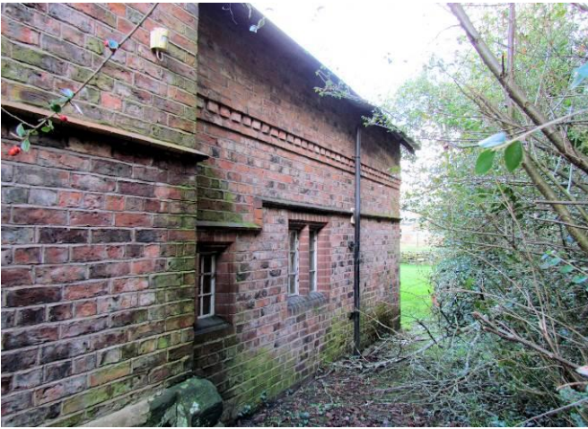
East Elevation of North Wing
