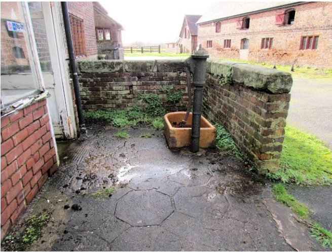
Brick Enclosure and Water Pump
