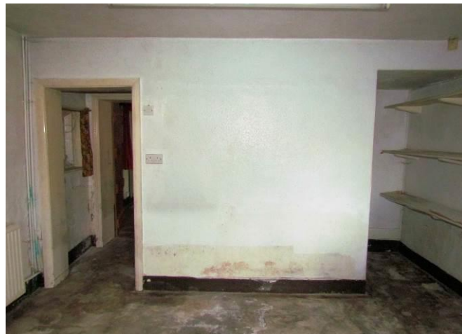
South Side of Kitchen
