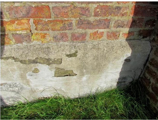
Surfacing on Plinth
