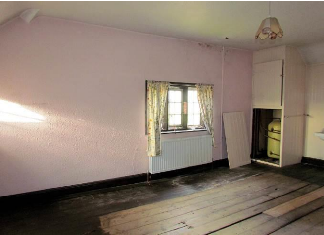
Western Room in Cross-wing
