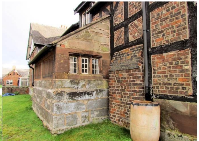
Detail of Buttress
