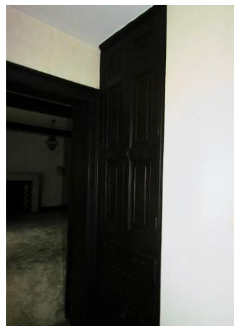
Cupboard in Stair Hall
