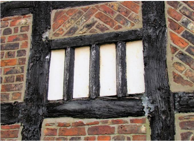
Detail of Timber-mullioned Window
