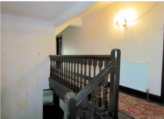
Top of Balustrade
