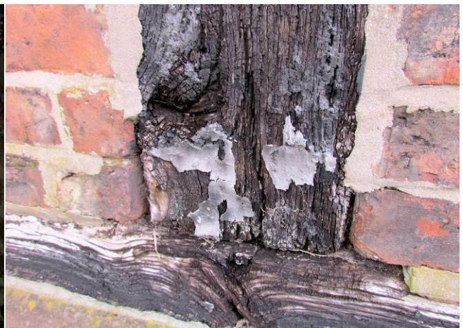
Cement Mortar in Timber-Frame
