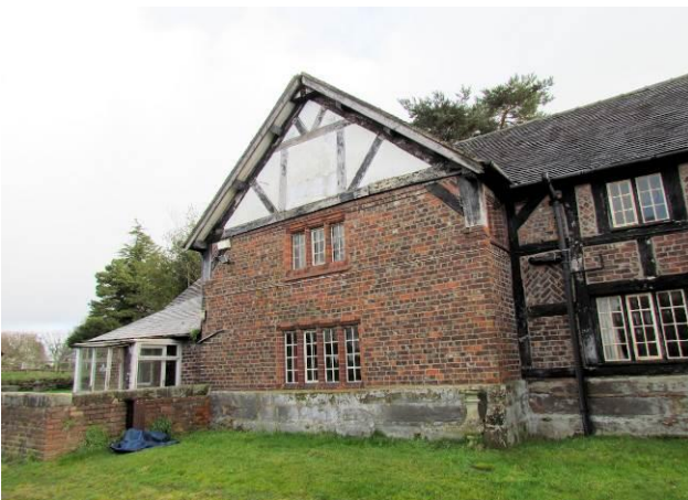
West Elevation of Cross-wing
