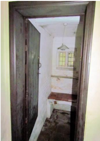
Access to Basement
