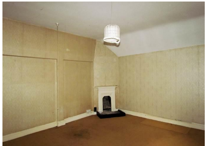
Eastern Room in Cross-wing
