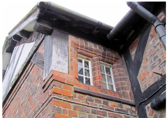
Detail of Replaced Post
