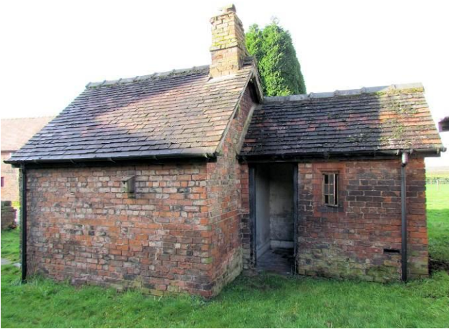
Toilet at Rear
