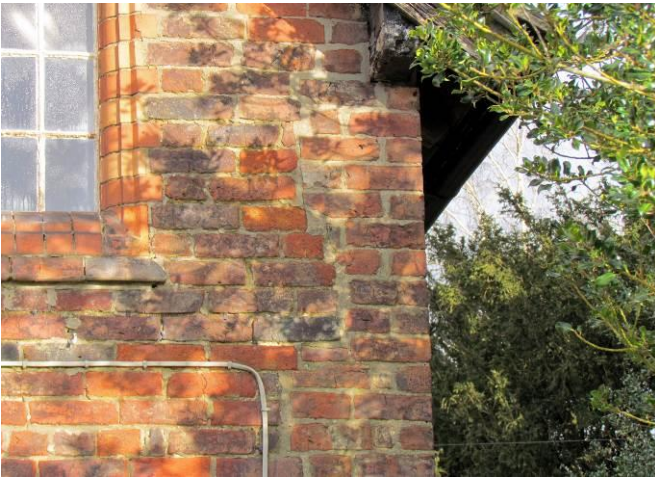
Line in Brickwork, South Elevation
