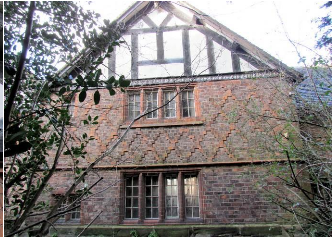
East Elevation of Crosswing, Bay 4
