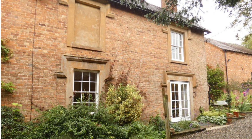
Site of proposed extension viewed from the south east
