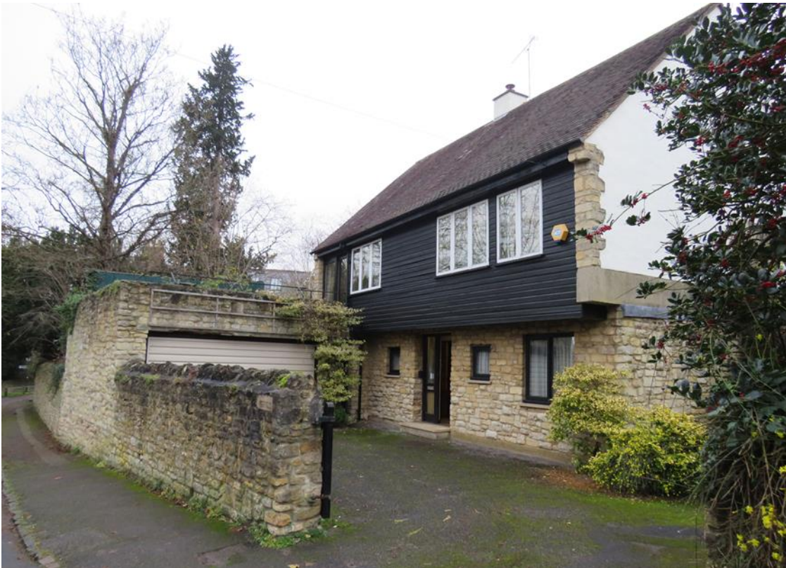
West elevation, from Mill Lane
