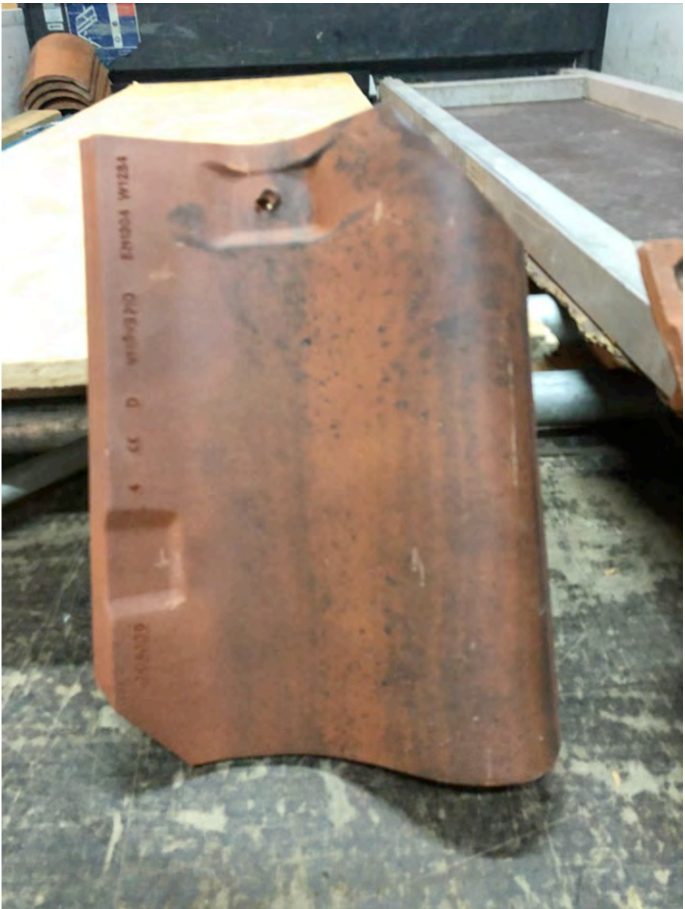
Roof pantiles: Sandtoft New Machine-made; Arcadia
