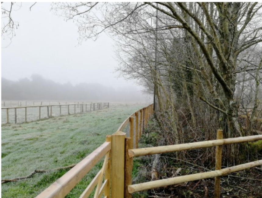
Figure 3. Photograph confirming that fencing has been erected adjacent to G2 and will delineate a construction exclusion zone.
