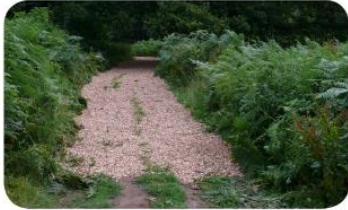
Step 1: Prepare Surface
