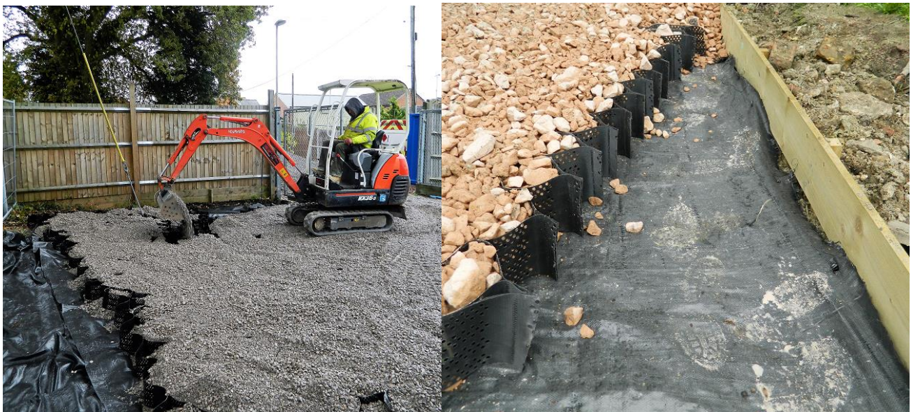
Figure 5. Photographs illustrating cellular confinement system used to form an above-ground no-dig surface.
