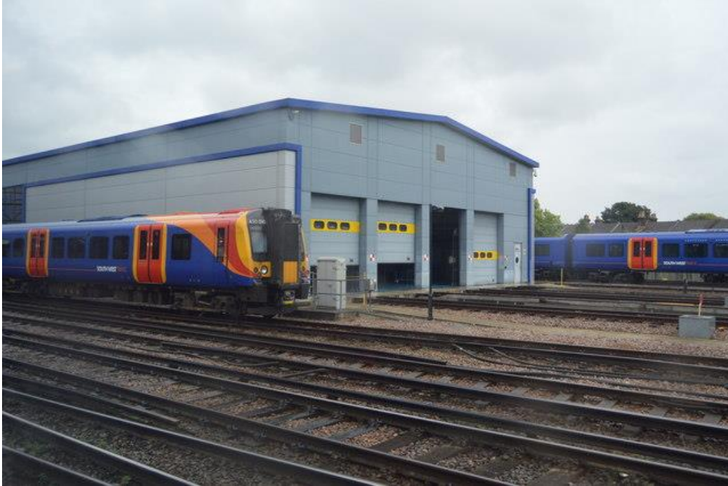
A maintenance shed at Northam train depot in Southampton
