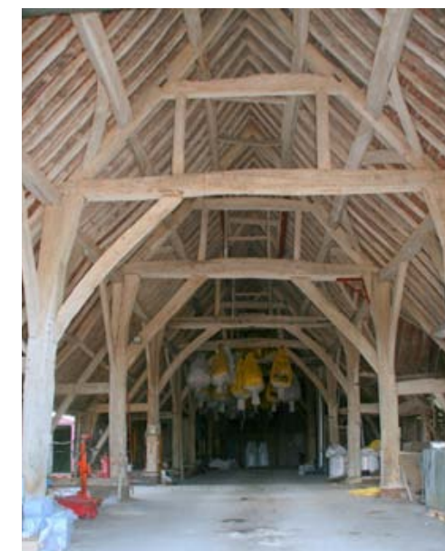
A handsome exposed oak aisle structure.
