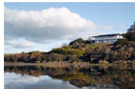
Sensitive approach to design within natural landscape setting, reduce negative effect on visual amenity.
