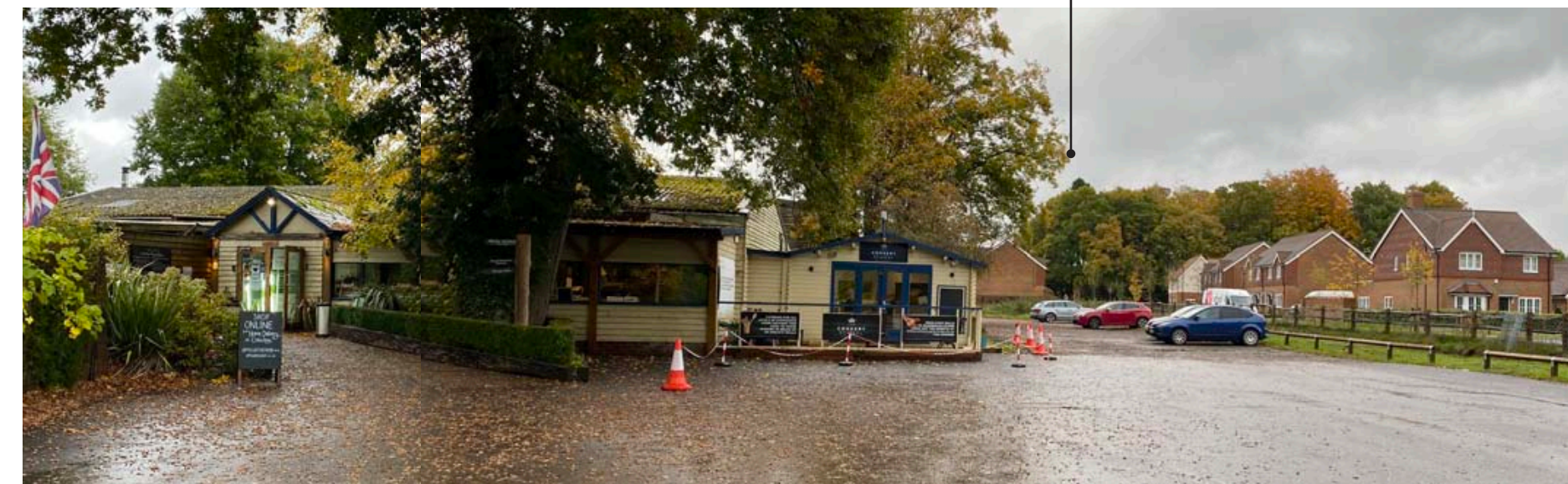
View of Applegarth site from the south - this will form one of the key vistas for the new building.
