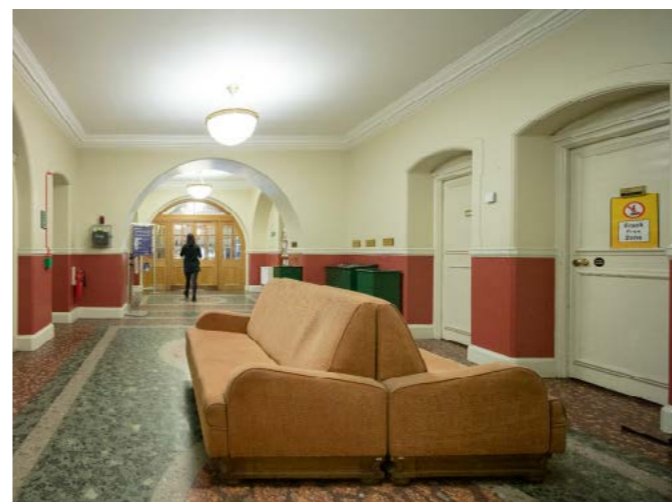
Original terrazzo flooring in entrance of Norman Shaw South
