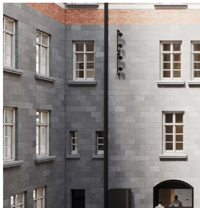
Montage showing same, shorter lighting bar co-located with rain water pipe
