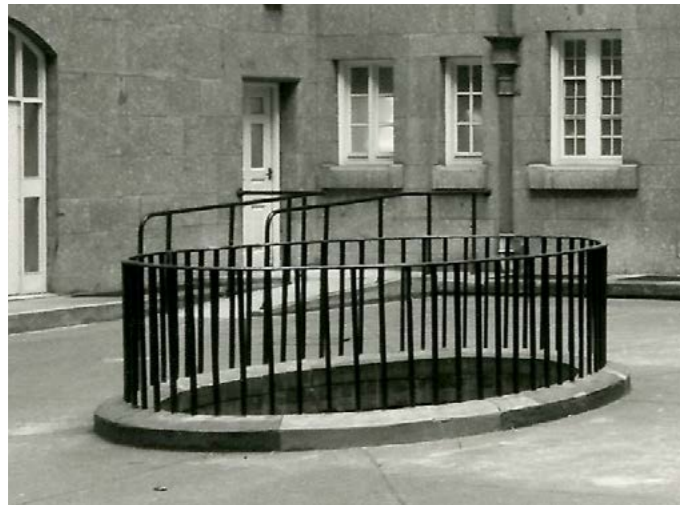
Photograph of oculus prior to removal and installation of portacabins
