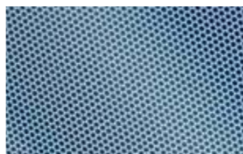
Double glazed panels with micro-dot ceramic frit for anti-slip to perimeter zone
