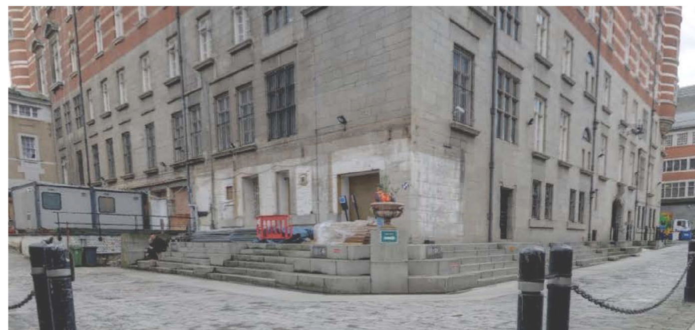
Photo of existing NW corner
