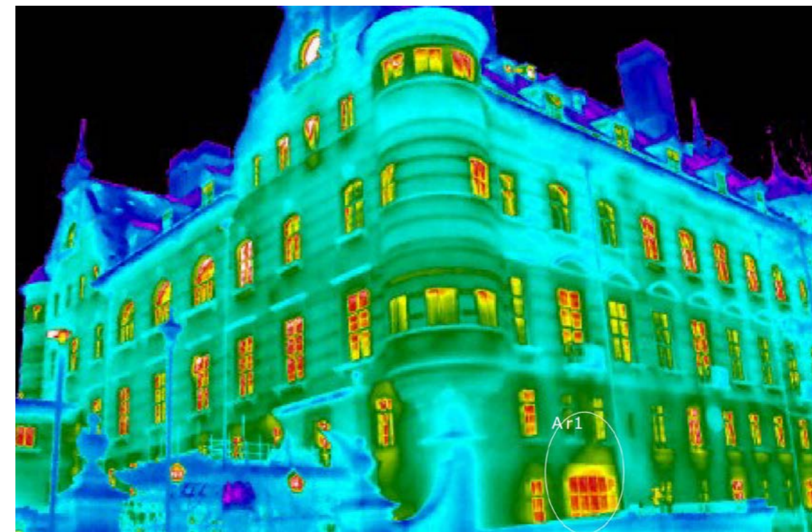
Thermal imaging highlighting opportunities for improvement at existing windows and the main roof that will be addressed in the proposals
