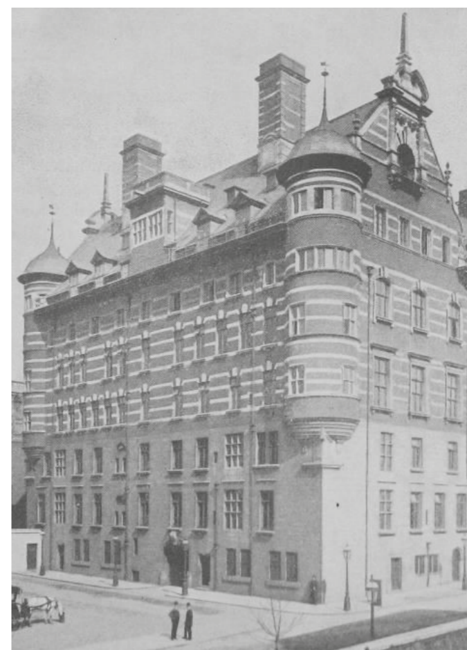
Early photo of NSN west facade showing landscape levels at or near plinth height.
