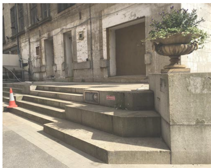
Photo of existing stepped plinth
