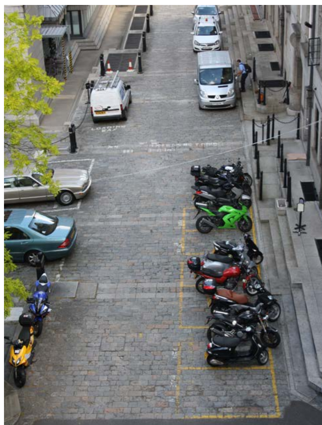
Whitfield paving design for Laundry Road, now removed and overlaid with asphalt
