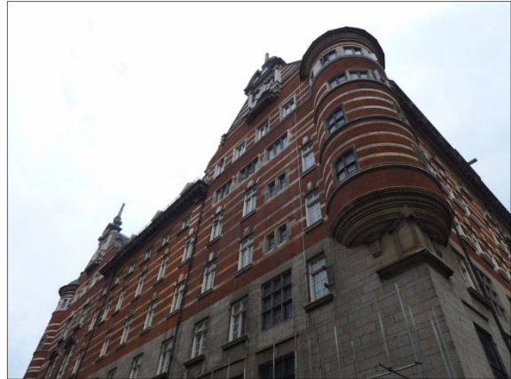
Plate 2. NSN (north-west elevation)
