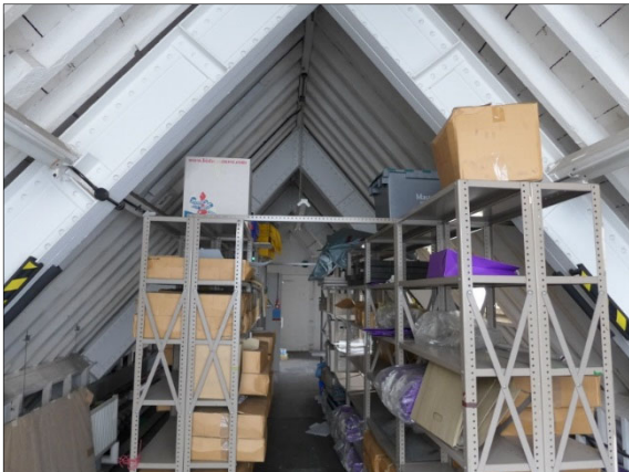
Plate 7. NSN internal roof space
