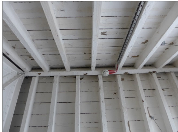
Plate 8. NSN internal roof space
