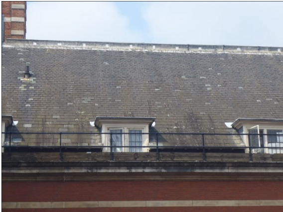
Plate 3. NSN slate roof covering
