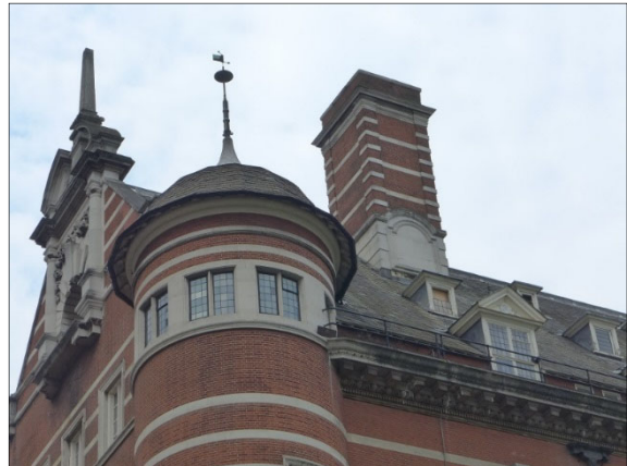
Plate 6. NSN conical roof on a cylindrical turret
