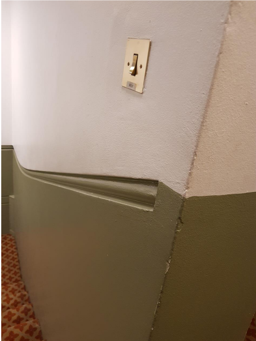
60. Bead to staircase GST2
