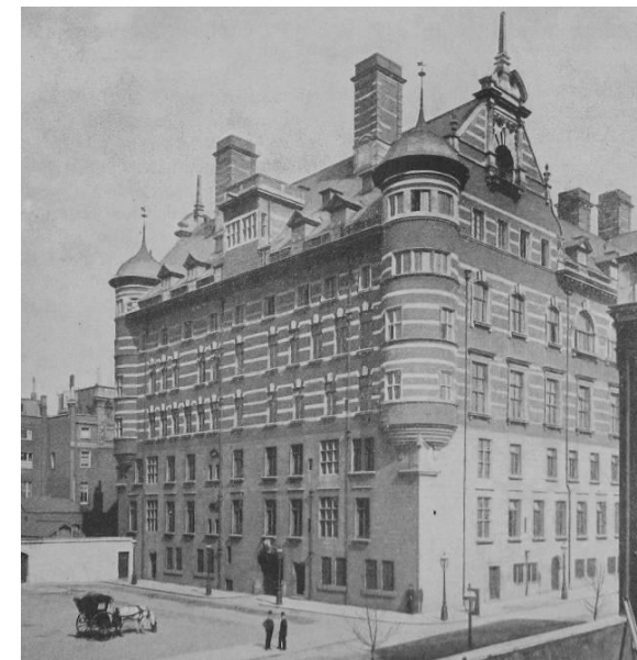
9b. Early photograph of west elevation
