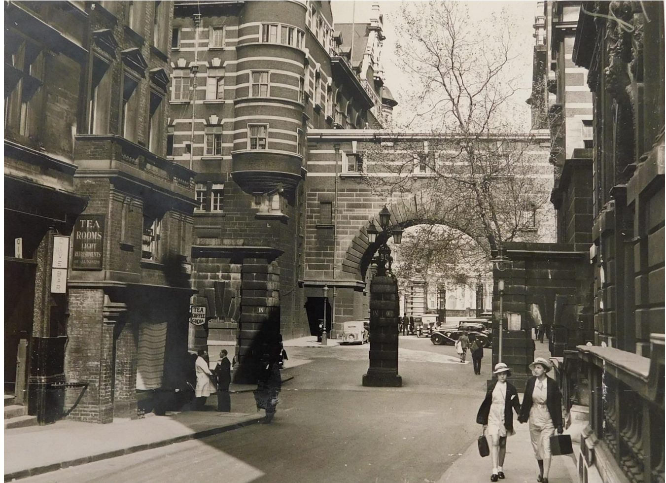
24. New Scotland Yard bridge looking east (London Metropolitan Archives)
