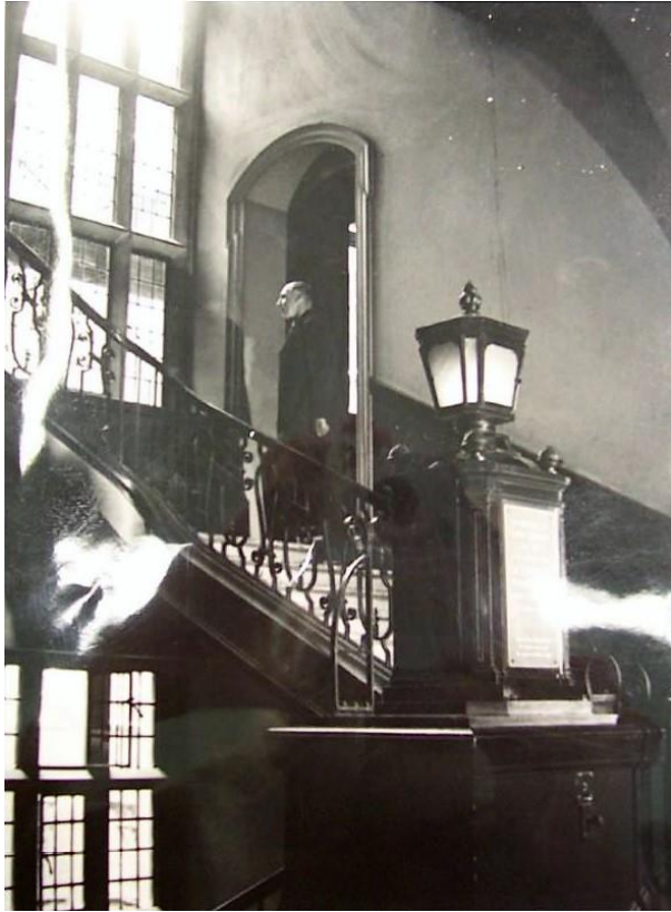
22a. Early photograph of principal staircase (National Archives)
