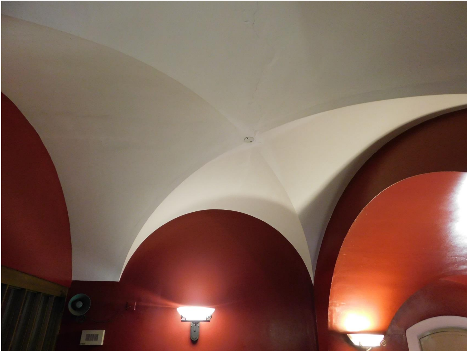
66. Cross vault to lobby of 1ST3
