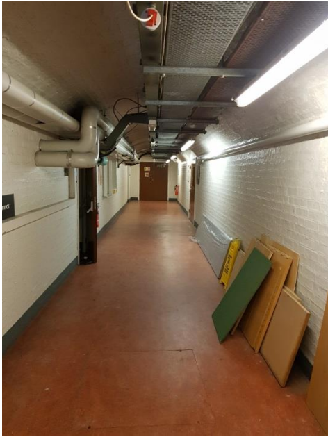
51. Corridor to basement
