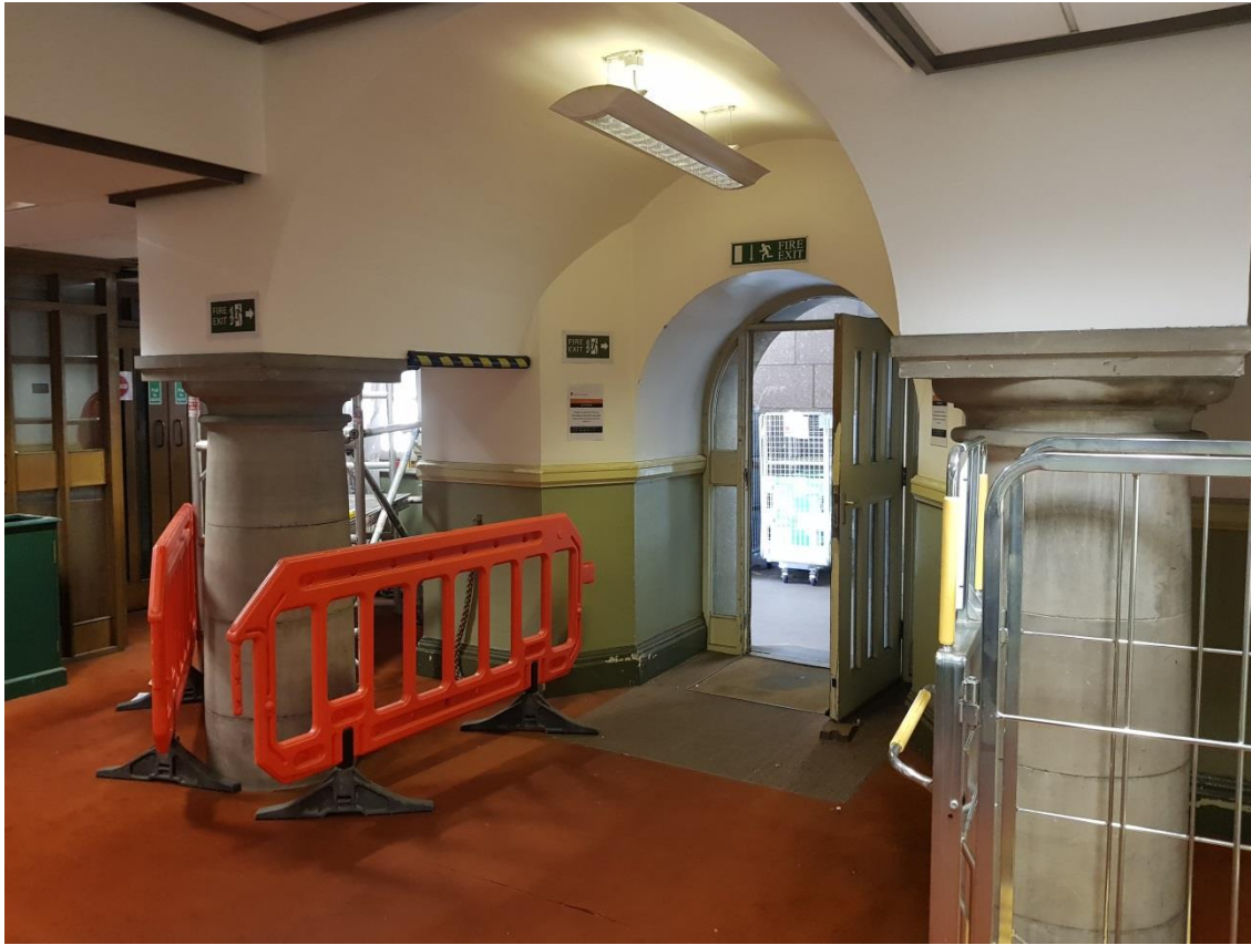
54. Squat Columns to LGC5
