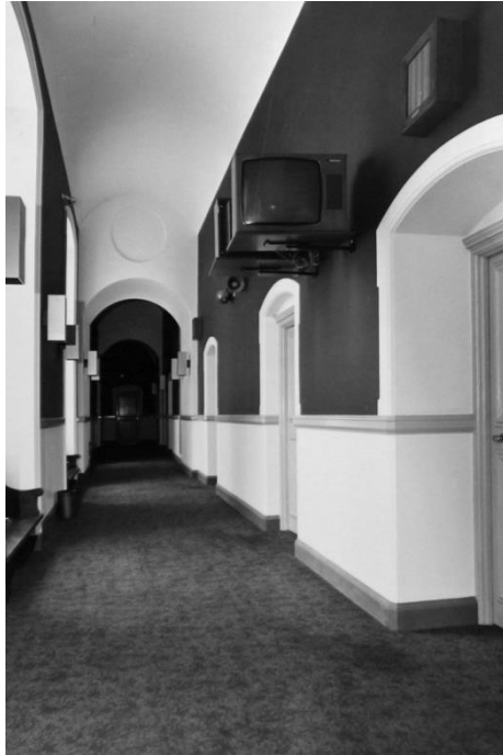
36d. 1975 corridor refurbishment (Parliamentary Archives)
