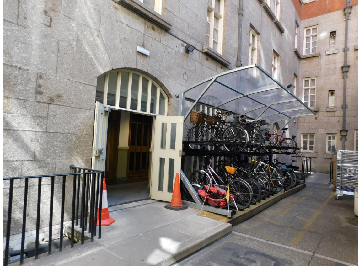
44. Modern doors to North Courtyard Elevation
