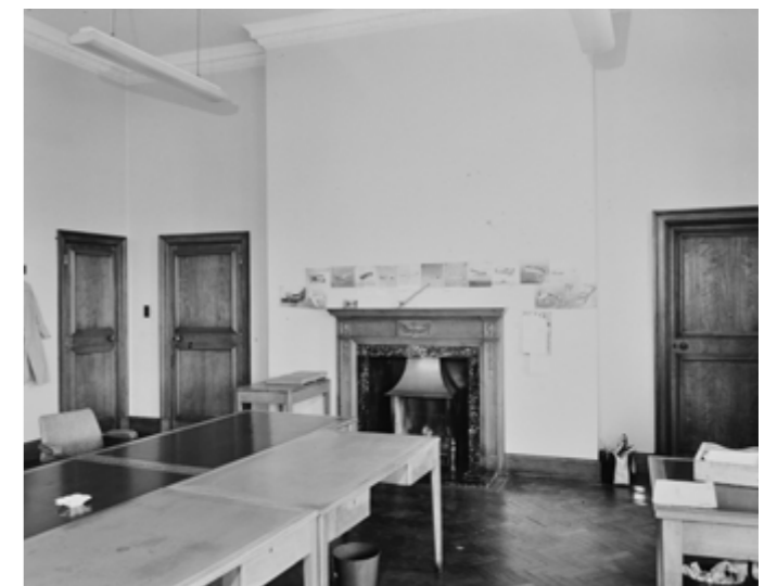
Commissioner's room entrance and chimney piece, 1970 (London Metropolitan Archives)
