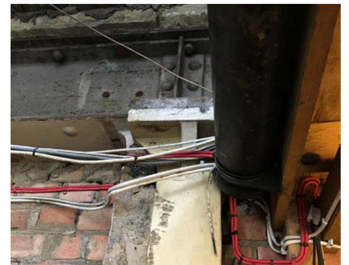
Existing condition of columns
