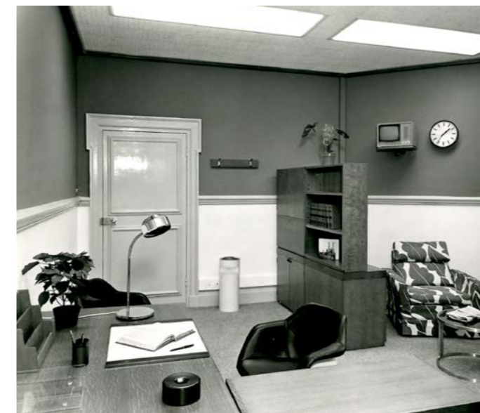
Typical office post 1970s refurbishment illustrating new suspended fabric ceilings, low level surface mounted trunking and new decorative finishes throughout
