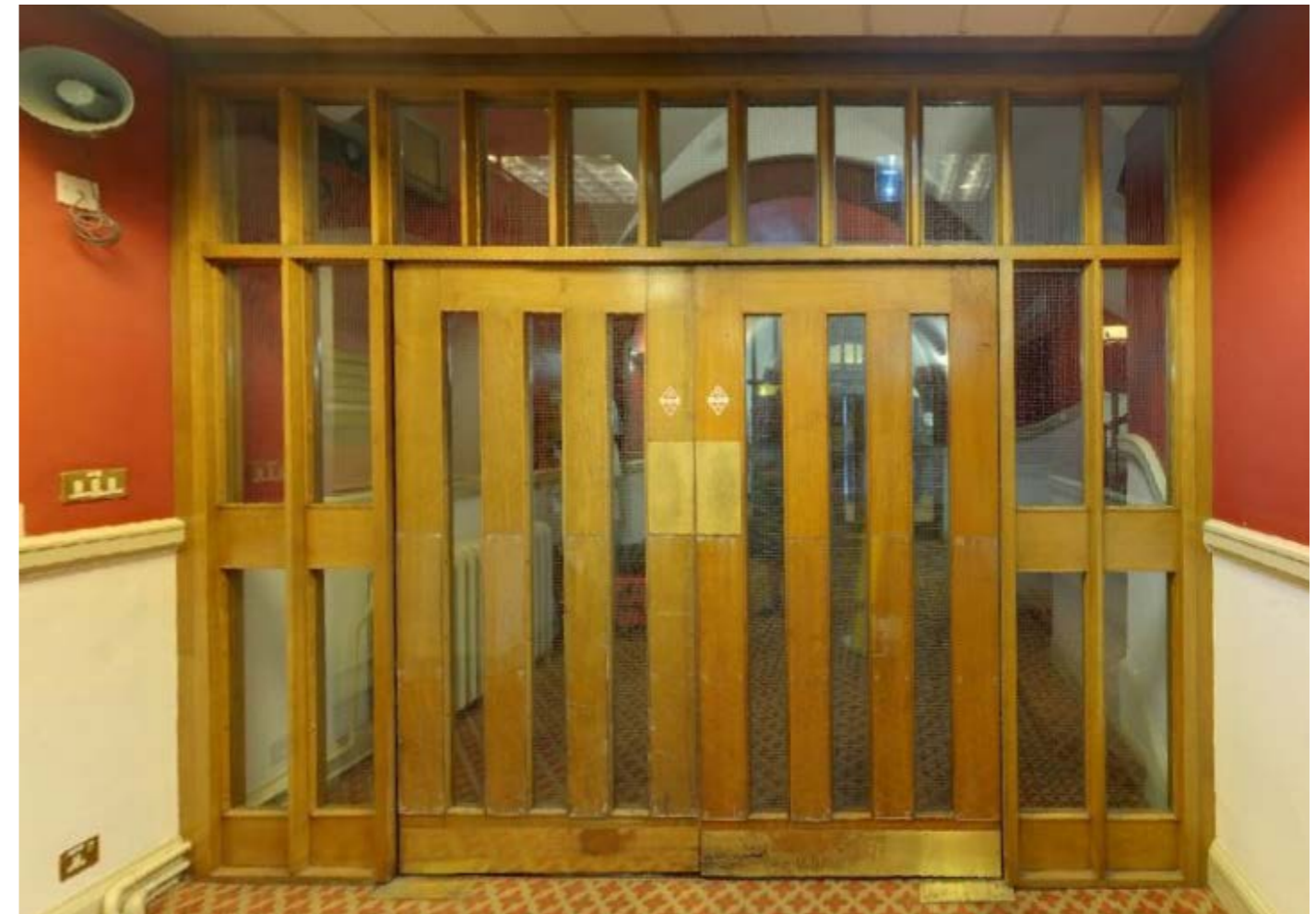
Existing timber cross corridor screen
