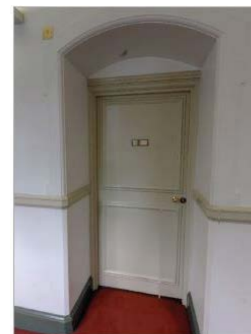
Office doors within Norman Shaw North
