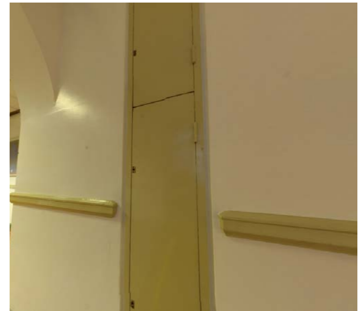
Example of joinery encasement in corridor containing rising electrical services.
