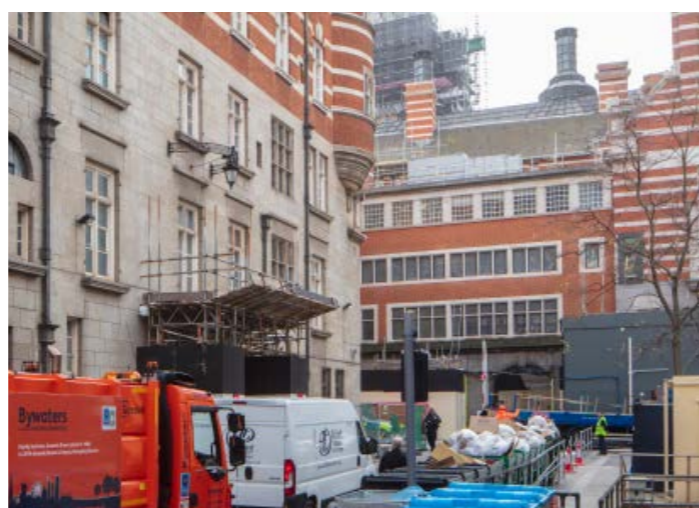
Laundry Road looking south
