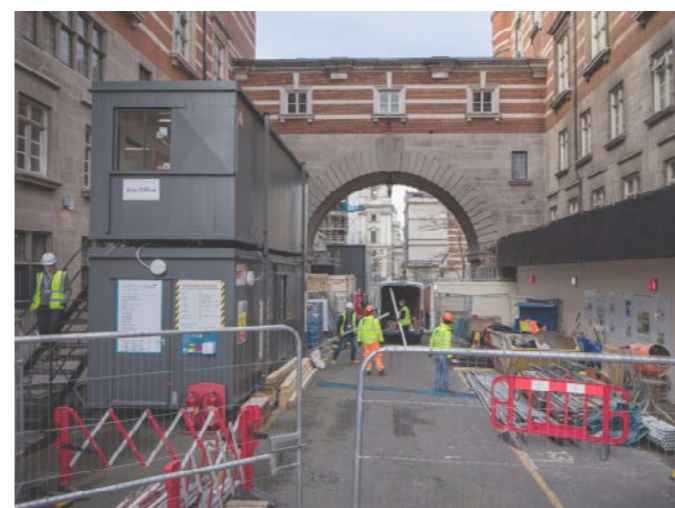
Commissioner's Yard looking west
