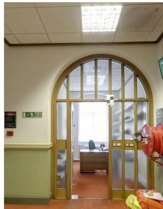
Fire doors obstruct views along corridors
