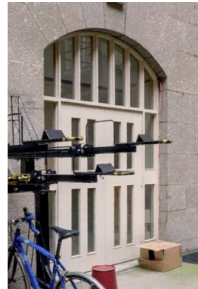
4 - Existing screens on north facade
