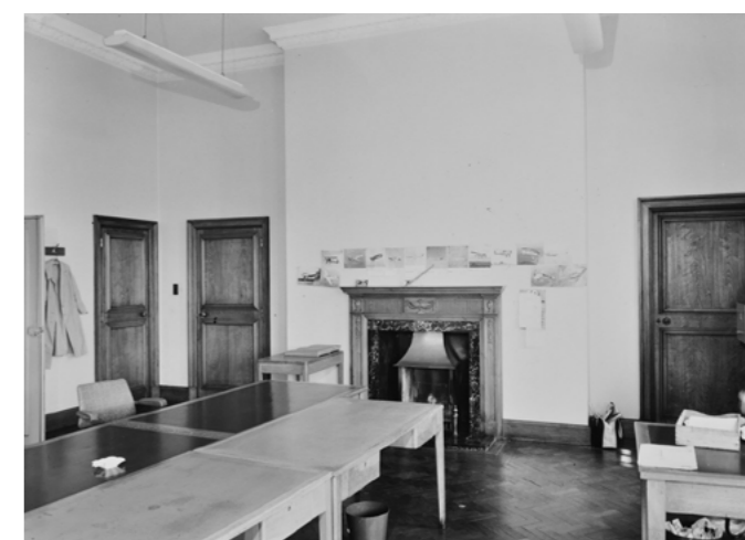
Commissioner's Room entrance, 1970 (London Metropolitan Archive) chimney piece and decorative skirtings, dado rails and plaster cornice
