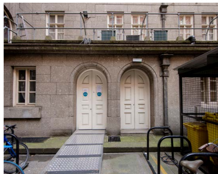
3 - Temporary ramp required for level access
