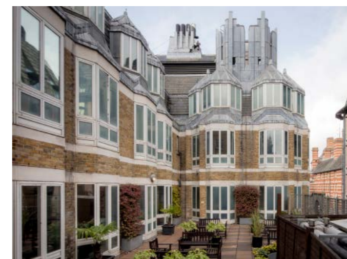
Upper levels of existing Parliament Street Buildings
