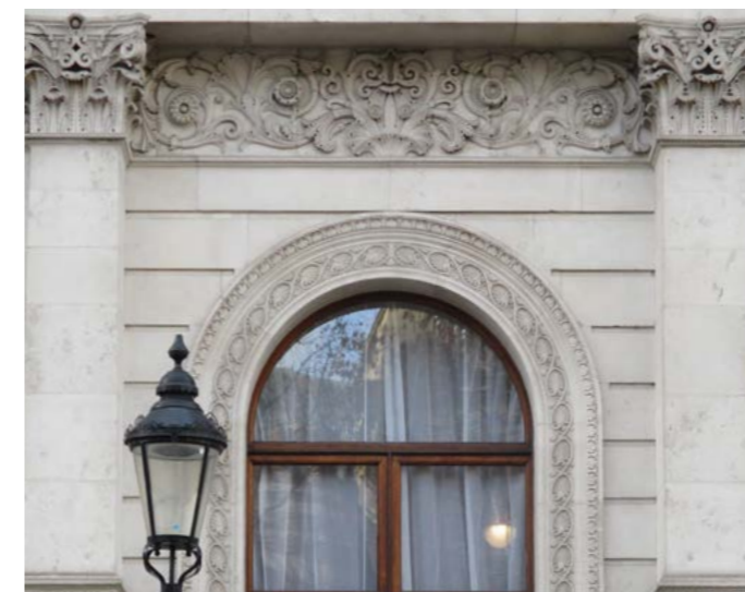
Facade detail of Foreign and Commonwealth building
