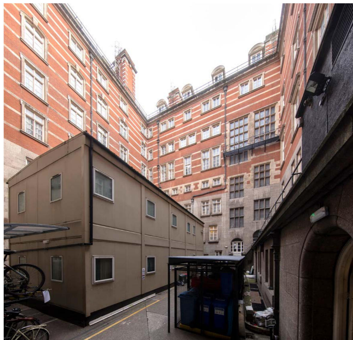
1 - Central oculus has been removed and space occupied by two storey portacabin
