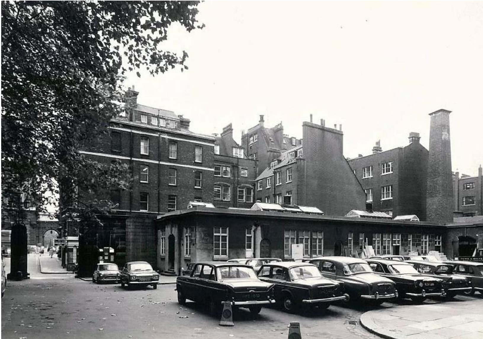
29. Laundry block with chimney, demolished 1975
