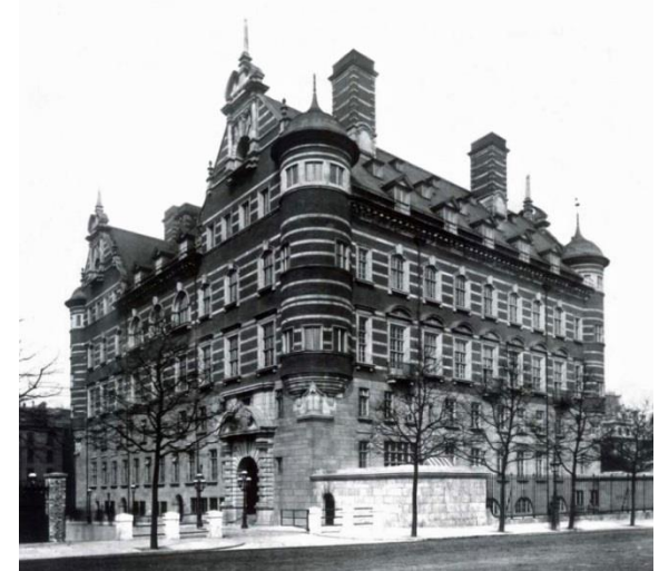
8b. East elevation and early railings, 1890 (London Metropolitan Archives)
