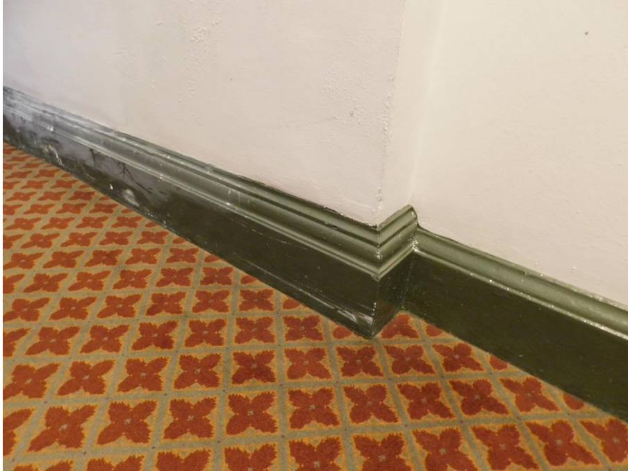
62. Two types of original skirting in 1C2
