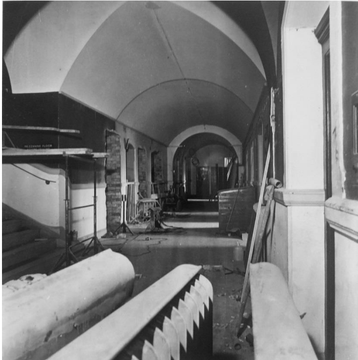
36a. 1970s corridor refurbishment in progress ( Architects Journal )
