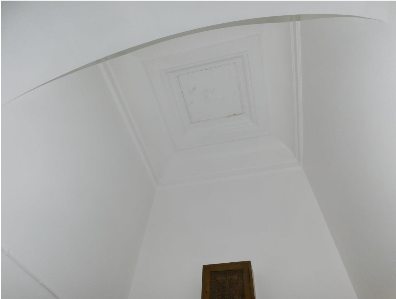
72 South lobby to 4C4
