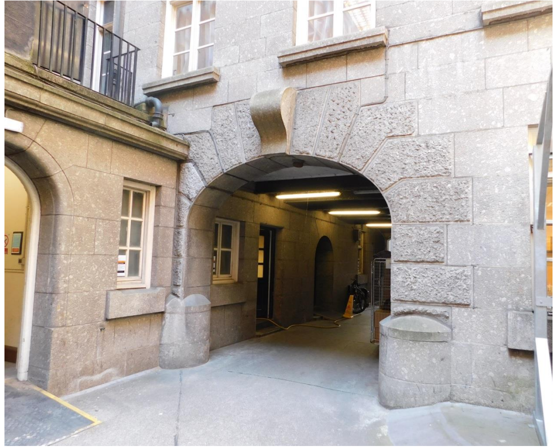
48. Original access passage to courtyard
