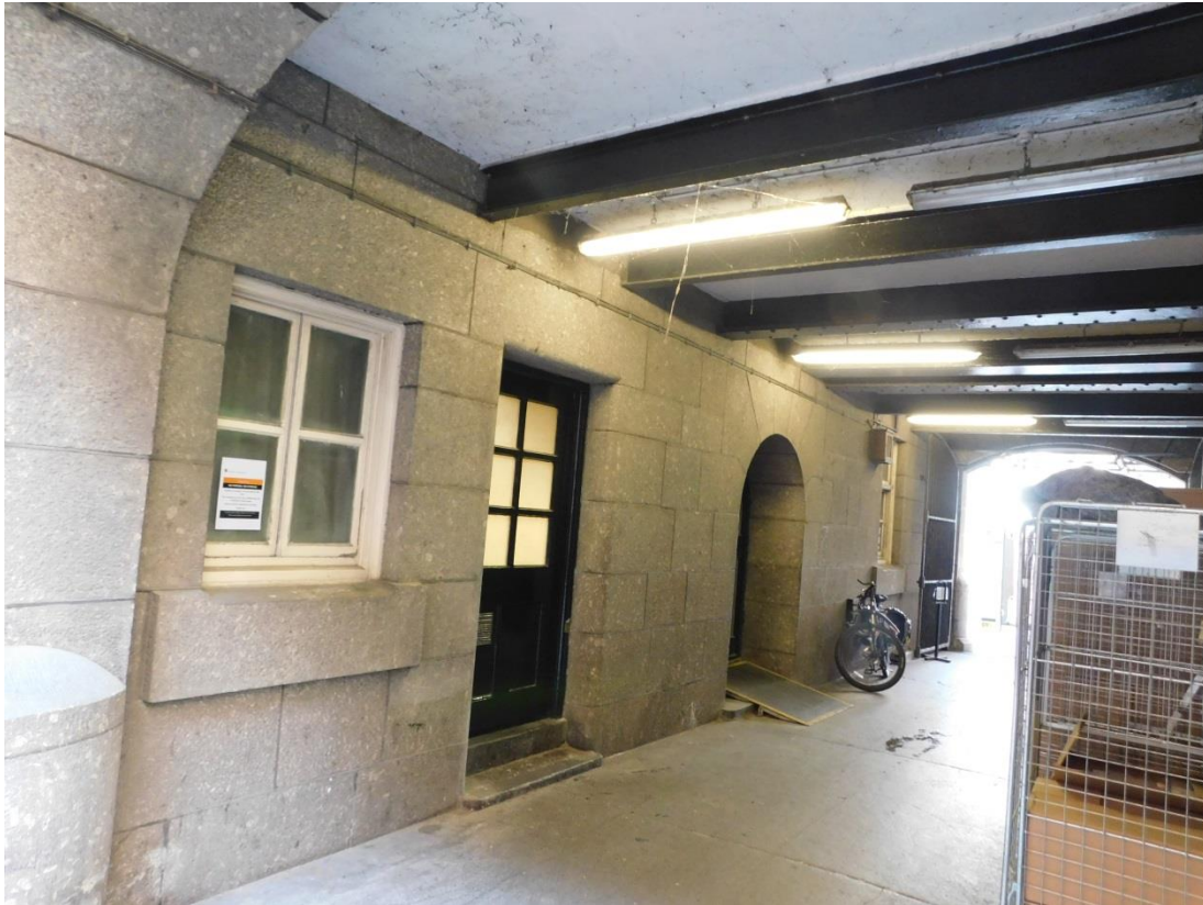
49. Original access passage to courtyard
