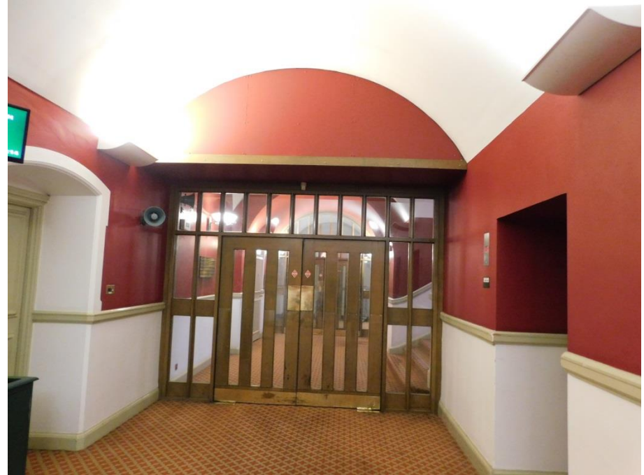
63. Infill to original barrel vault to 1C3
