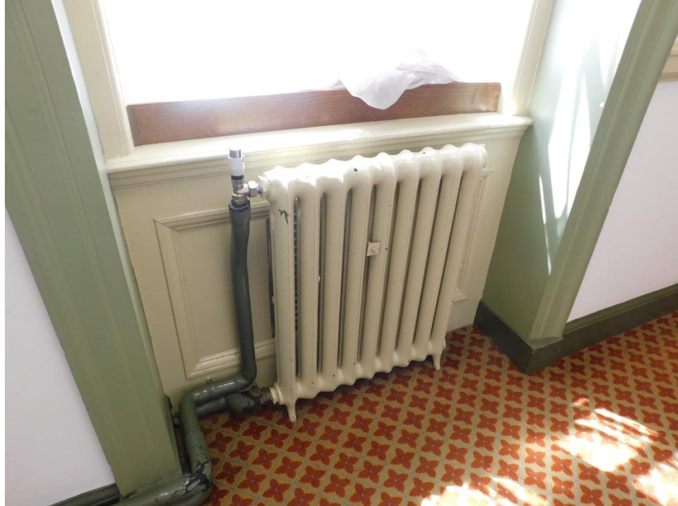
71. Original timber apron
