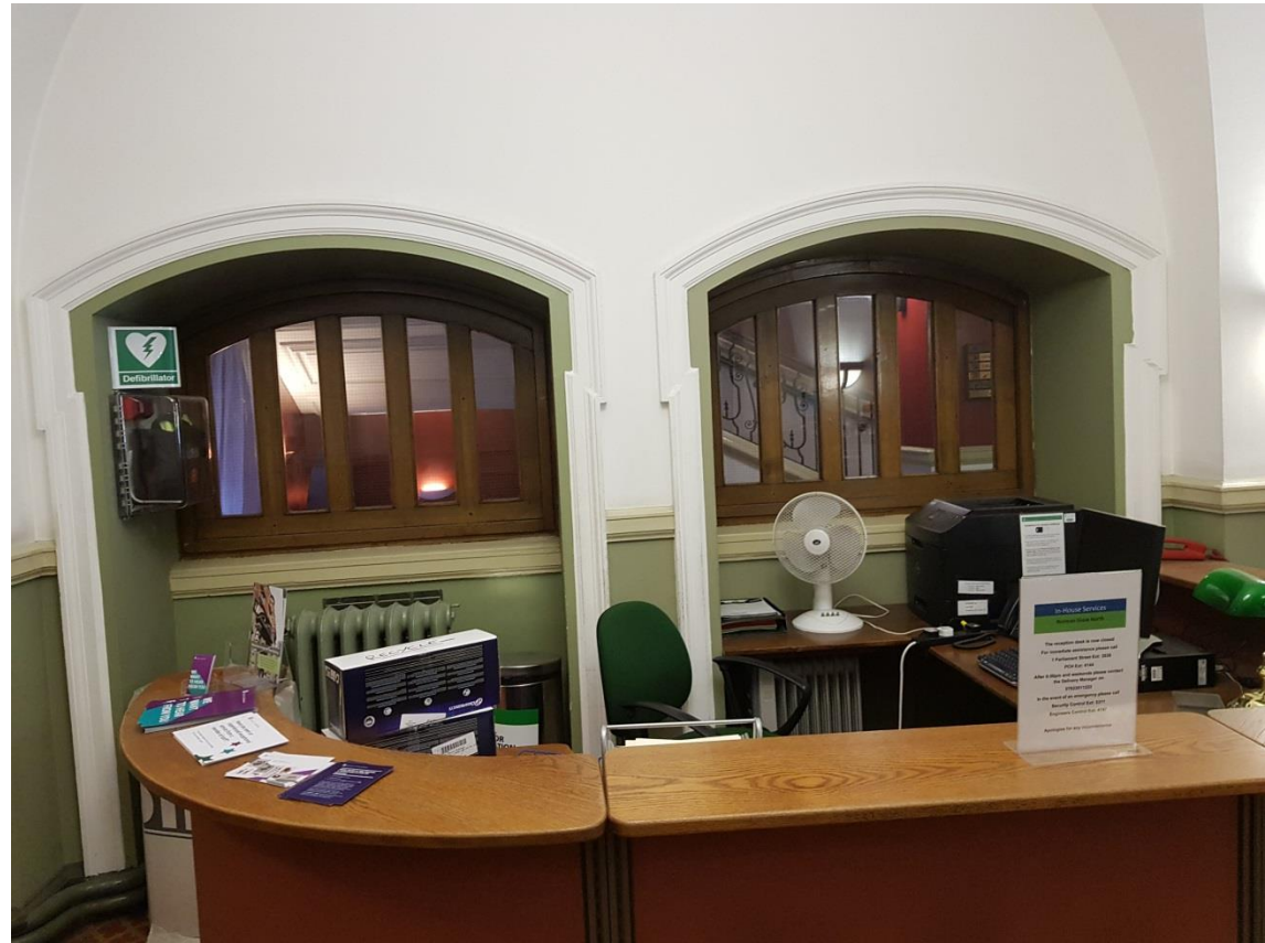
59. Original openings to the north elevation of GC4 with modern infill
