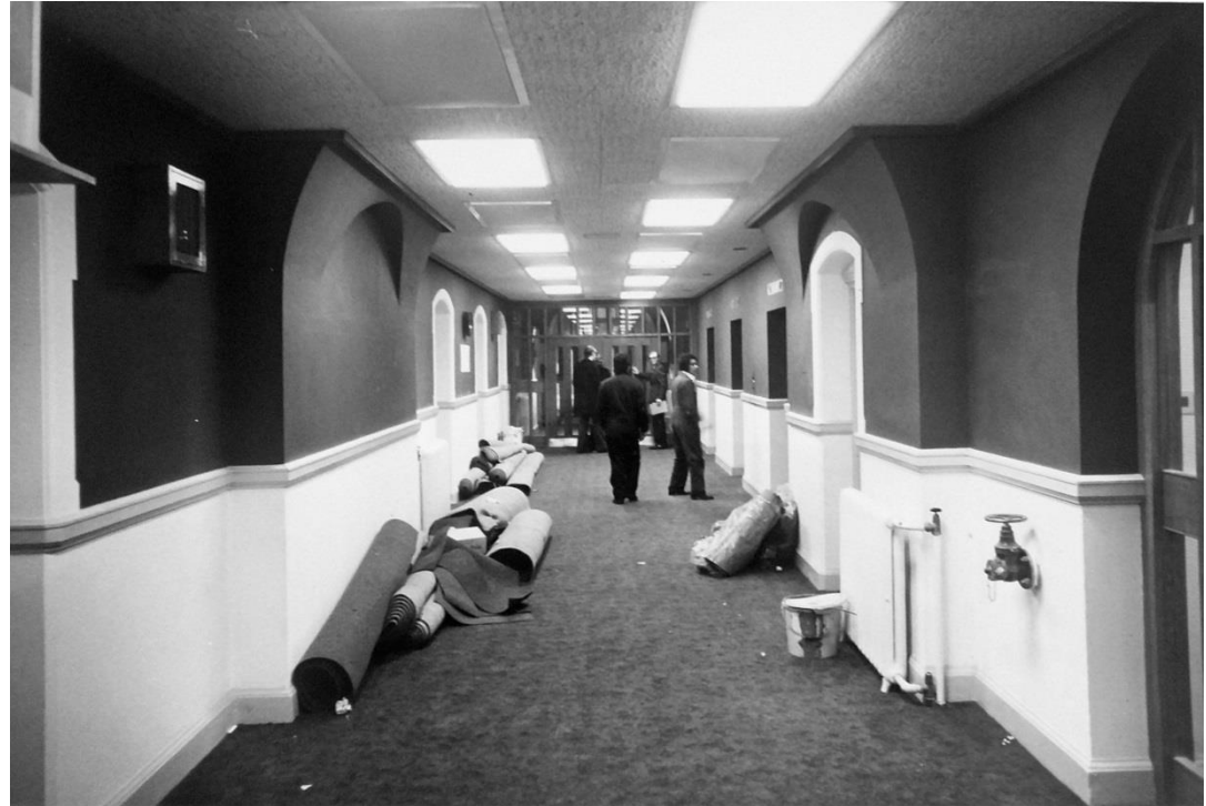
36b. Corridor refurbishment, 1975 ( Architects Journal )
