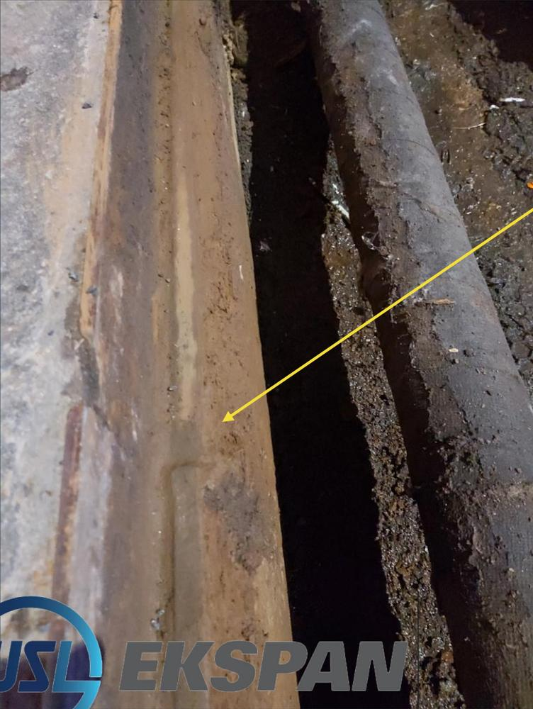
Slight high spots noted where existing bearing frame Sections meet each other
