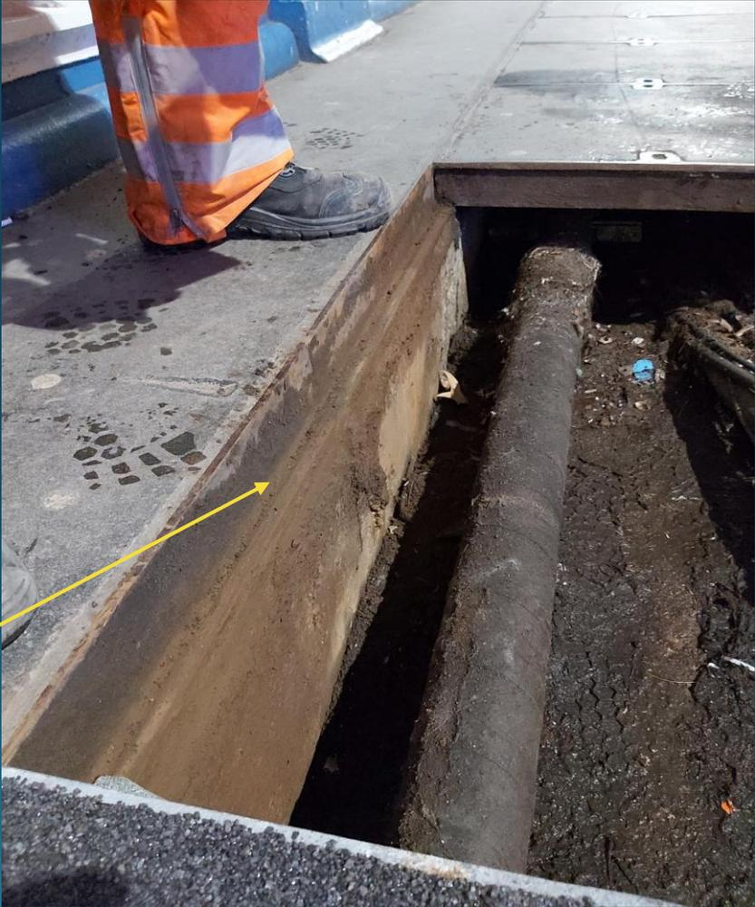
Bearing frame cleaned and prepared for new covers
