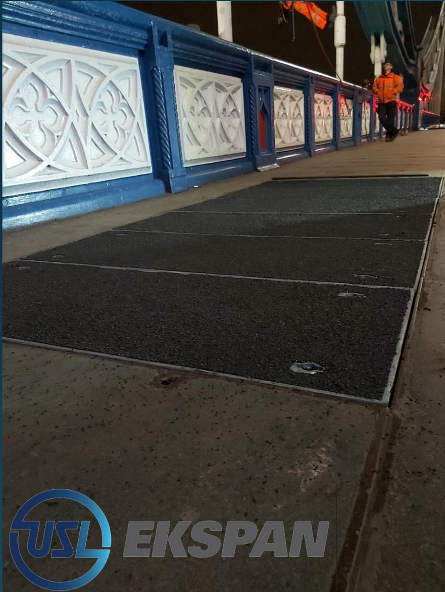
During the design period a request was made for the new covers to be Hot dip galvanised, this was carried out for the trial covers.
