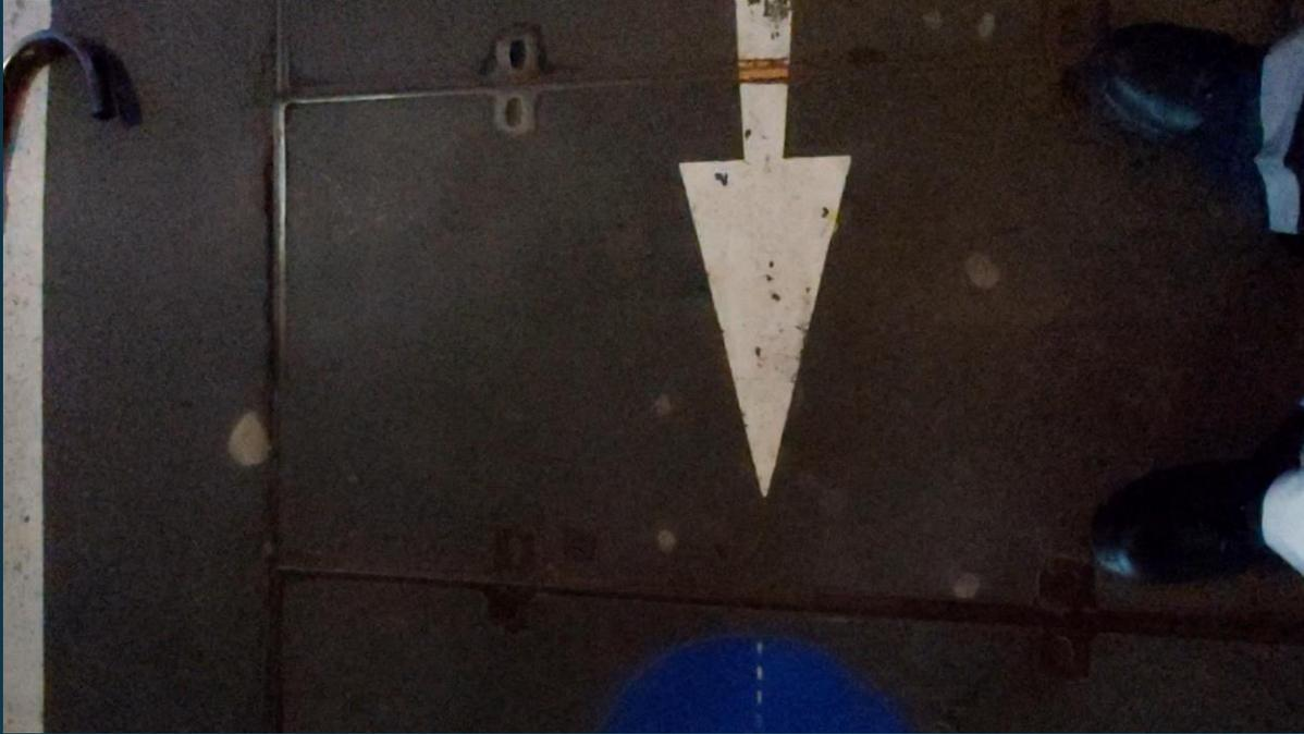
The “high spots” highlighted at the bearing frame joints is actually causing some of the existing covers to rock slightly.
