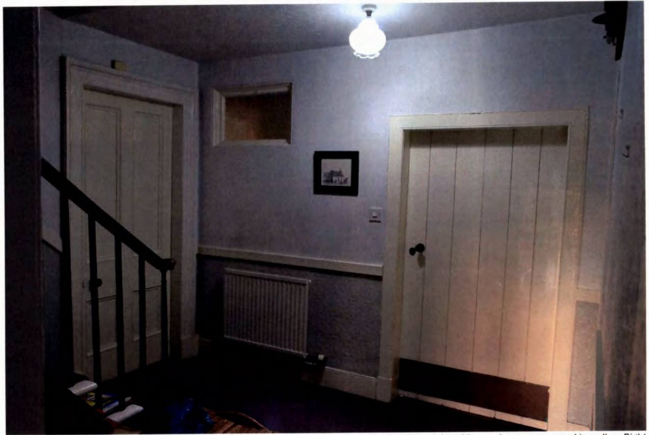
Photo of Existing Rear Hall showing various doors, apertures, ceiling heights, stairs with new doorway proposed in wall on Right
