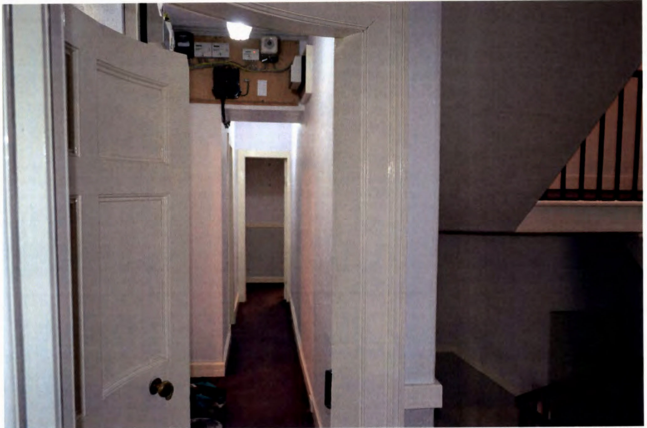
Photo of view of First Floor connecting corridor [to be blocked]
