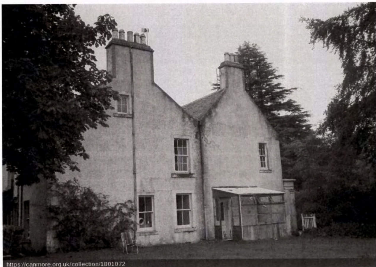
https://canmore.org.uk/collection/1801072 1983 West Side Elevation to garden with Greenhouse + Doorway
