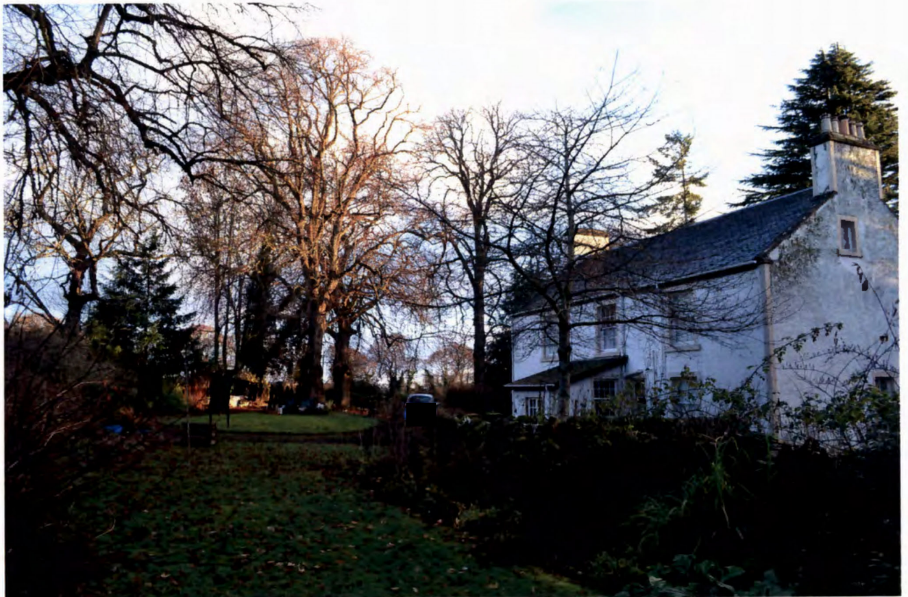
Photo of the rear of Wardlaw House
