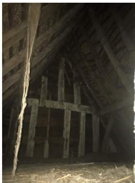
Fig 3 – View of timber roof structure
