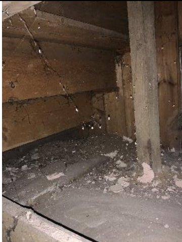
Brick floor and historic timber plate
