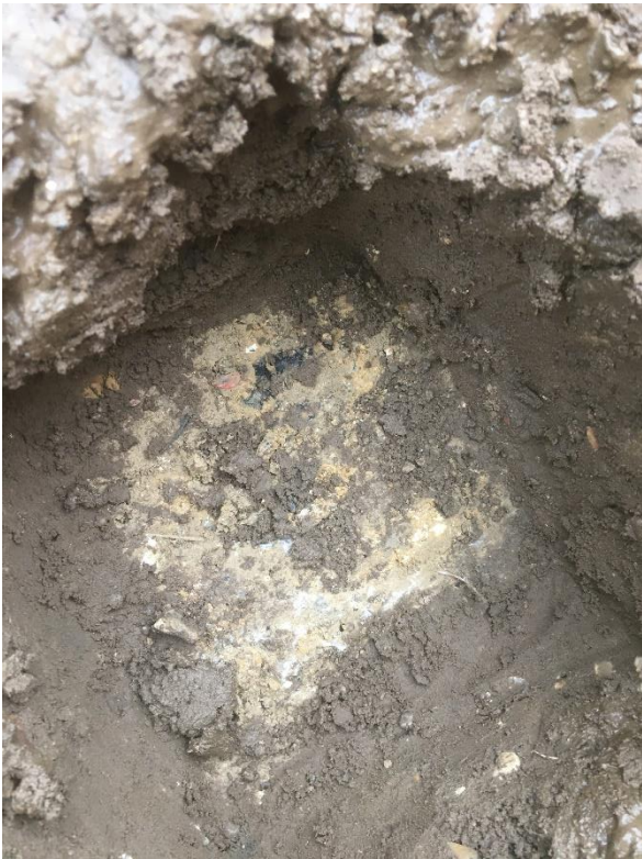
Photograph 7 , taken on the 15 th February 2021 showing the Concrete apron encountered within HDTP31-03.
